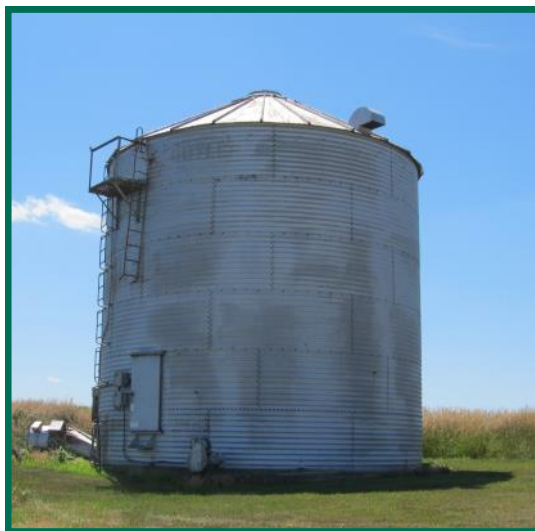
Parcel 2 - 9,000 bushel grain bin with aeration.
