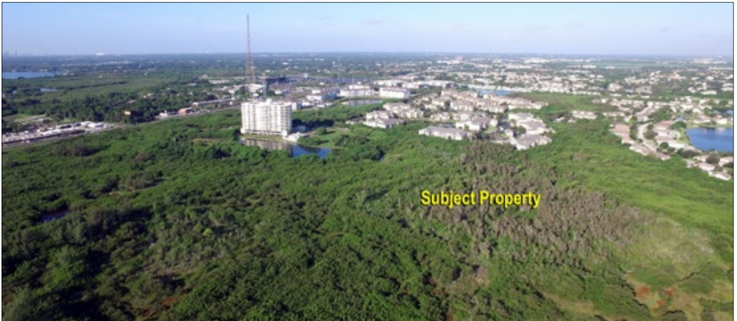
Looking West from Property
