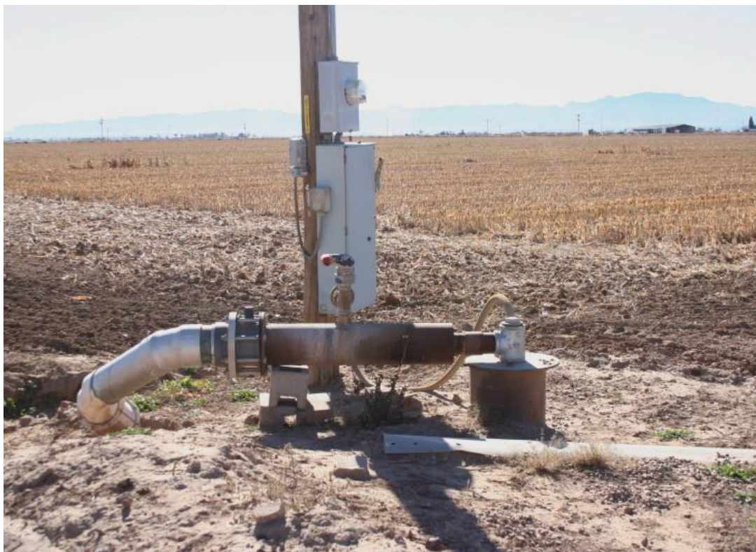
Well no. 2B, 147' deep, 20Hp, submersible, 400 GPM
