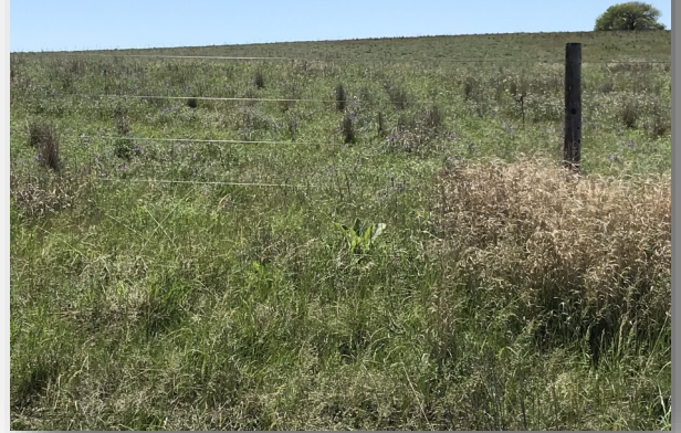
4-wire high tensile wire fence along the county roads
