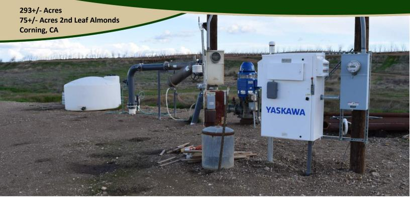
Well is equipped with variable speed drive motor and a spin clean filter.
