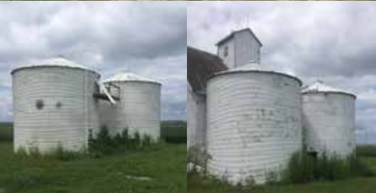
4 grain bins – All are 6 rings high with 16 Ft. Diameters.
