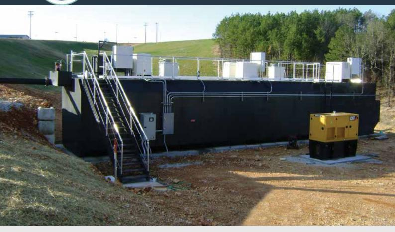
Tipton packaged wastewater treatments plants are customizable, simple to operate, and cost effective
