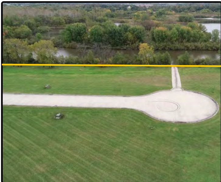
Parcel 1 - Cul-De-Sac and Boat Ramp
