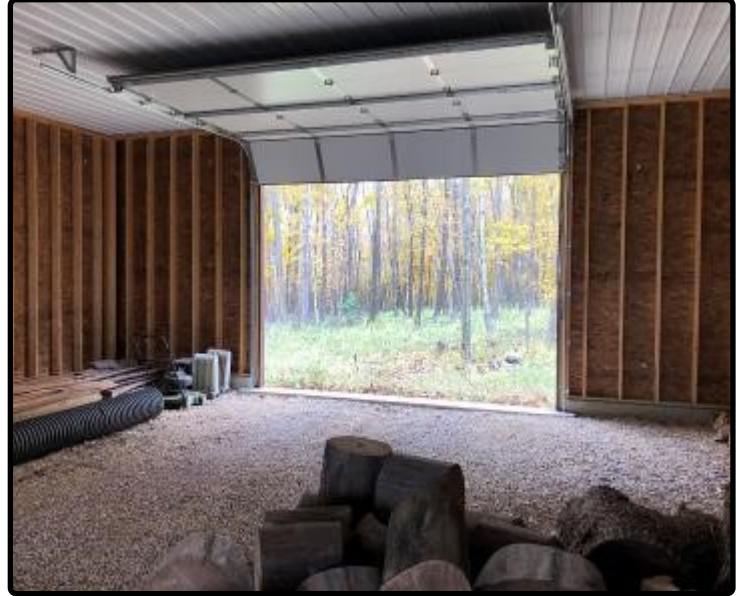
Shop - Large Overhead Doors
