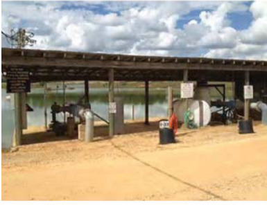
PUMP HOUSE (W/FERTILIZER INJECTOR)-RCP2
