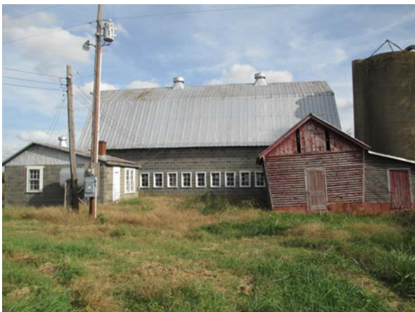
DAIRY BARN WITH SUPPORT BUILDINGS AND SHEDS
