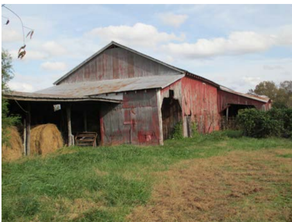
POLE BARN WITH EQUIPMENT LEAN-TOS
