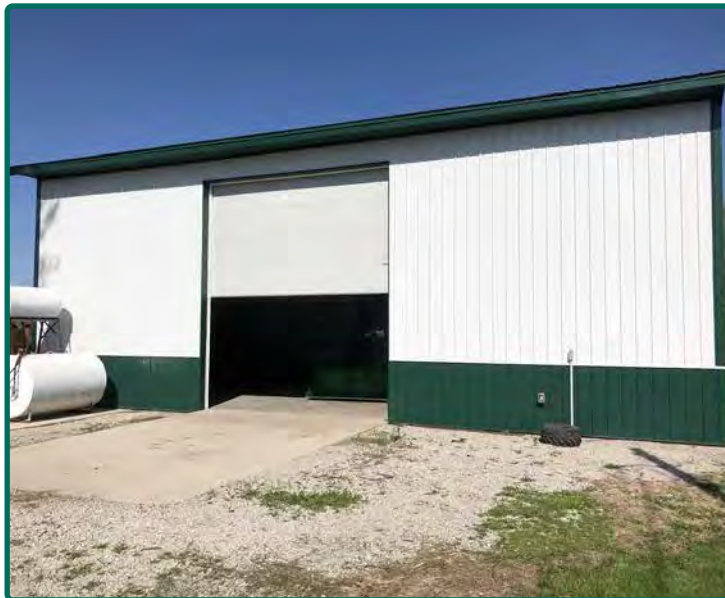
Steel Pole Shed w/ Concrete Floor
