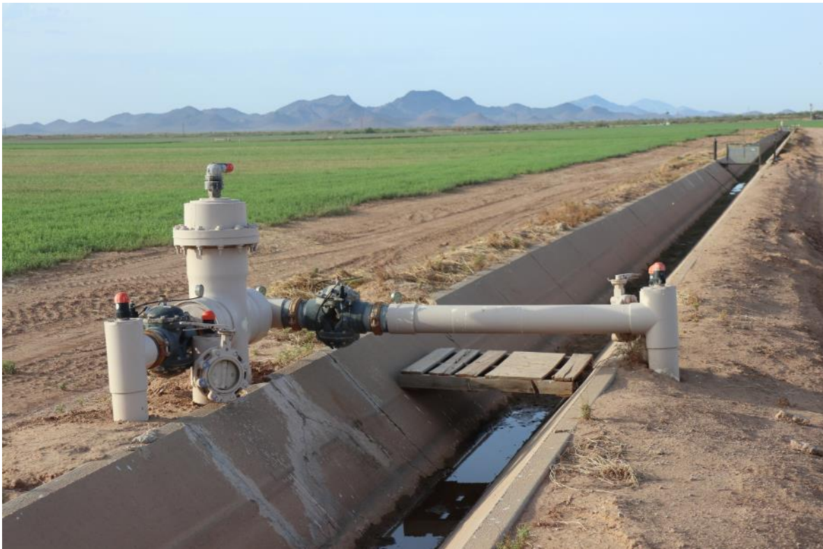
Drip irrigation valve system and concrete ditch
