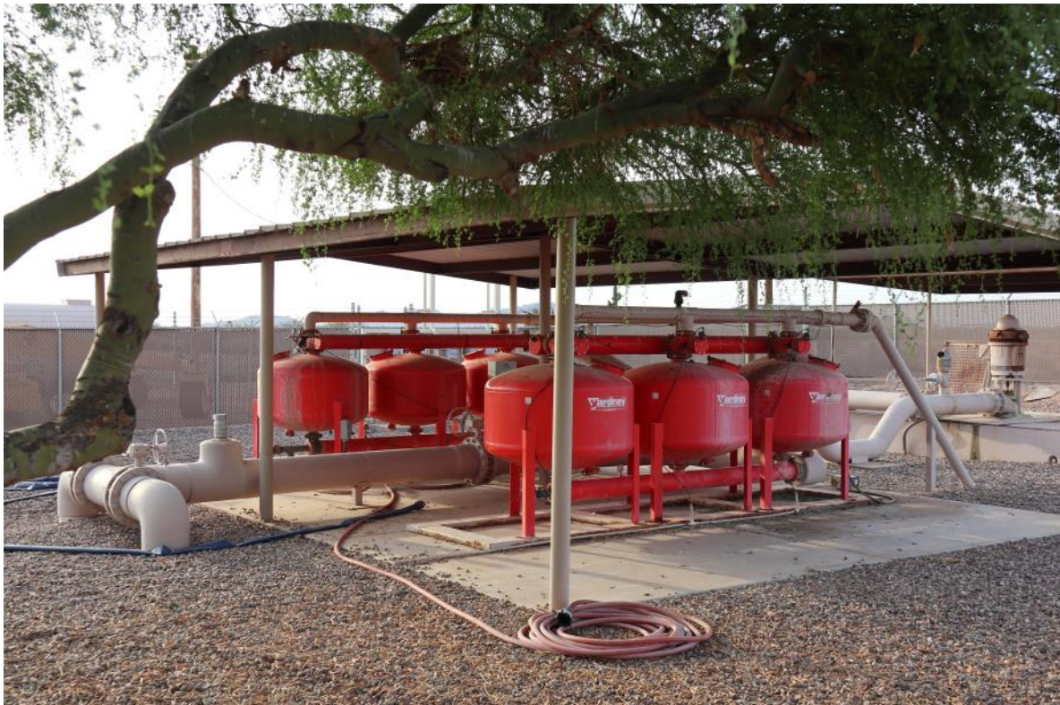
Drip irrigation sand media filters
