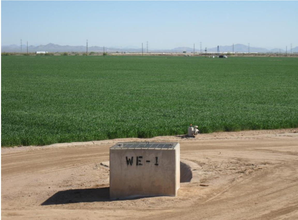
MSIDD irrigation water turn-out
