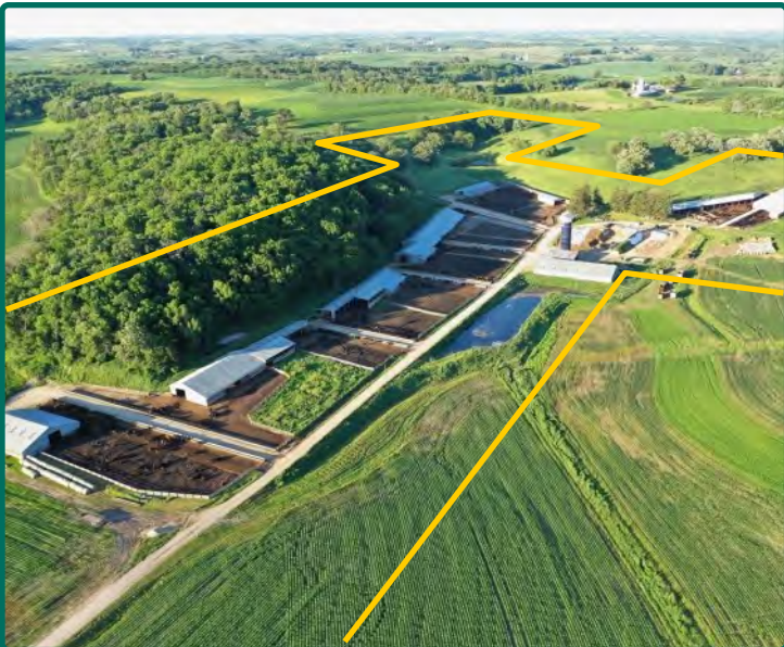
Cattle facilities—Looking northeast
