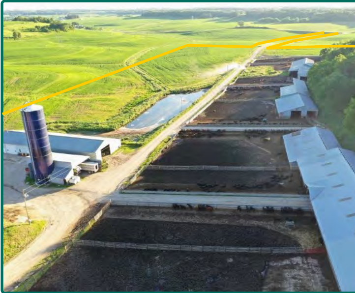
Cattle facilities—Looking west
