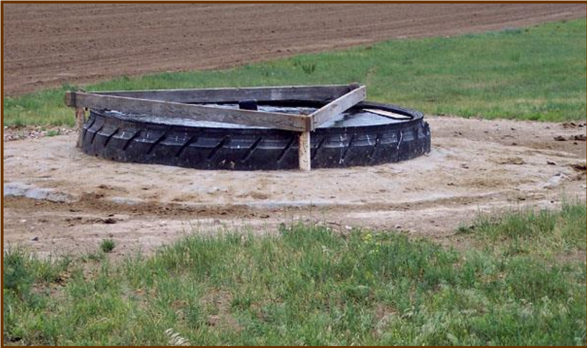
Both bottomless tanks connected to the underground pipeline have concrete aprons and float systems.
