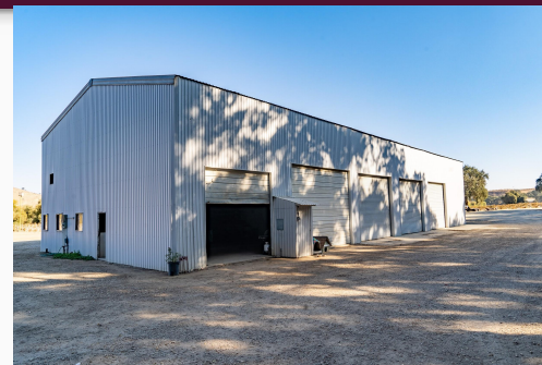
Shop with office and studio apartment located near Block 10
