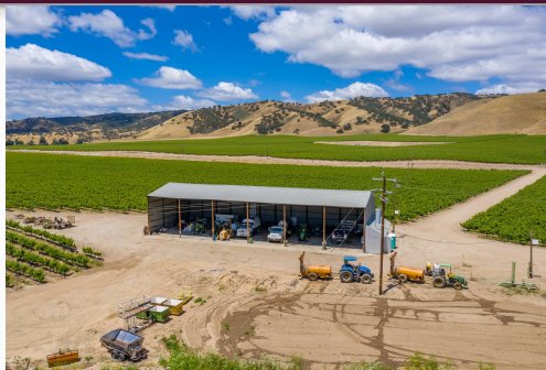
Equipment Storage Barn located in Block 2C
