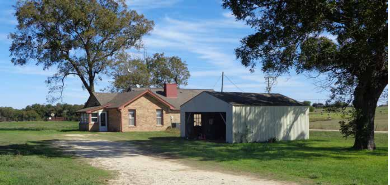
A rectangular 20'x25' (500 SF) garage/carport built with a concrete slab foundation, metal siding exterior and a composition shingle roof is located near the second house.
