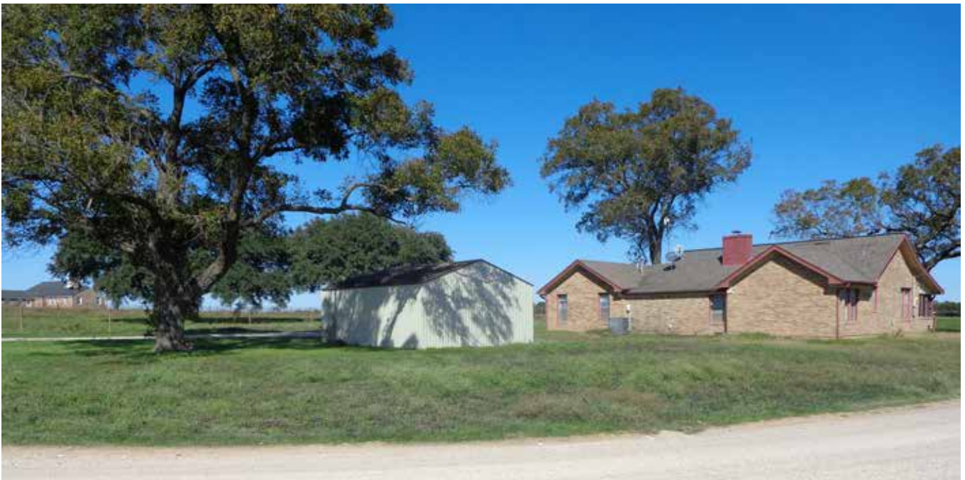
A rectangular 20'x25' (500 SF) garage/carport built with a concrete slab foundation, metal siding exterior and a composition shingle roof is located near the second house.
