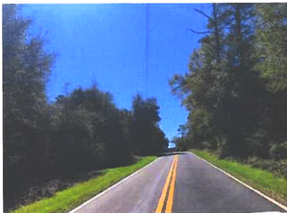
VIEW OF MORRISTOWN ROAD FACING SOUTH
