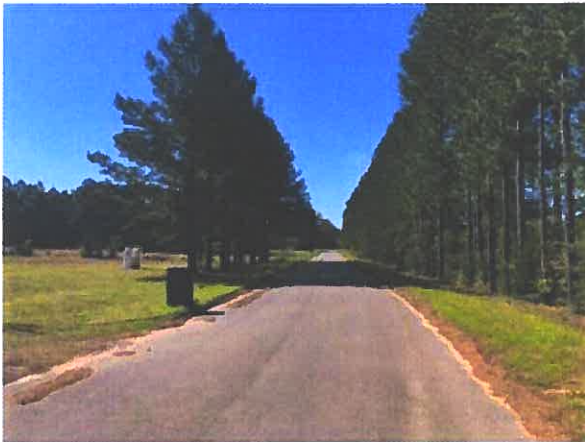
VIEW OF JOHN LOWERY ROAD FACING NORTH
