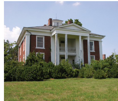
After years of deterioration
