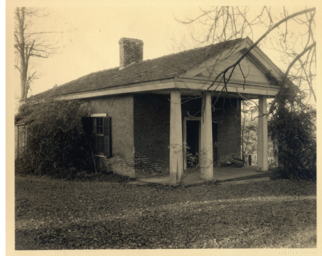
The building east of the house prior to being stuccoed.
