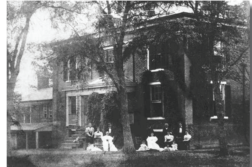
The rear view showing the original back porch
