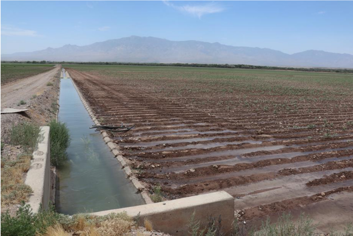
Notched concrete ditch
