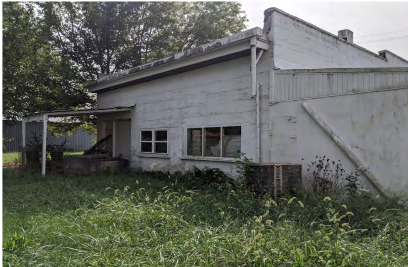
Photo 3. View of the on-site structure, facing southeast.
