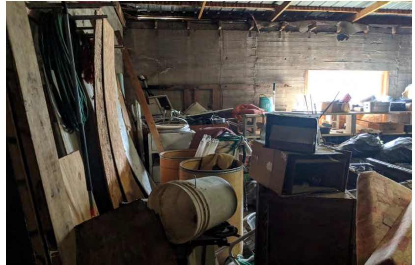
Photo 32. General view of the storage addition.
