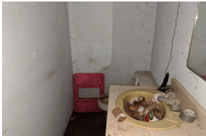
Photo 28. View of bathroom.
