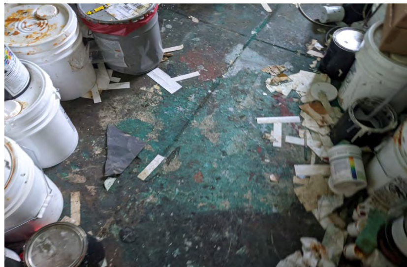
Photo 20. View of paint staining on the floor of paint equipment room.
