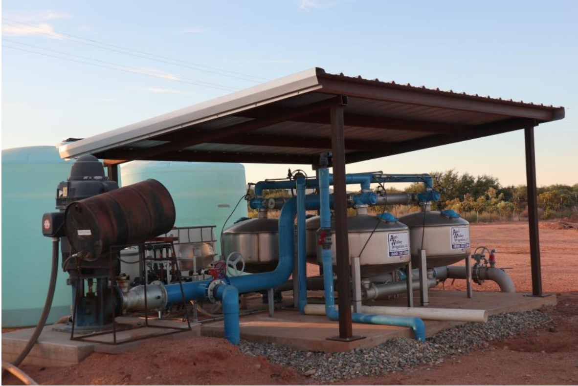
Well A, 1000' deep, static 260', 150 hp, 1000 GPM, with automated irrigation and chemigation system
