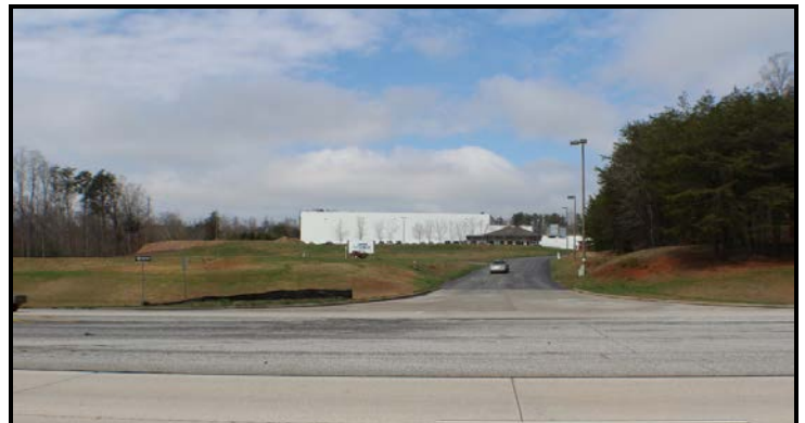
View of Lanier Cold Storage From Hwy 365 Frontage
