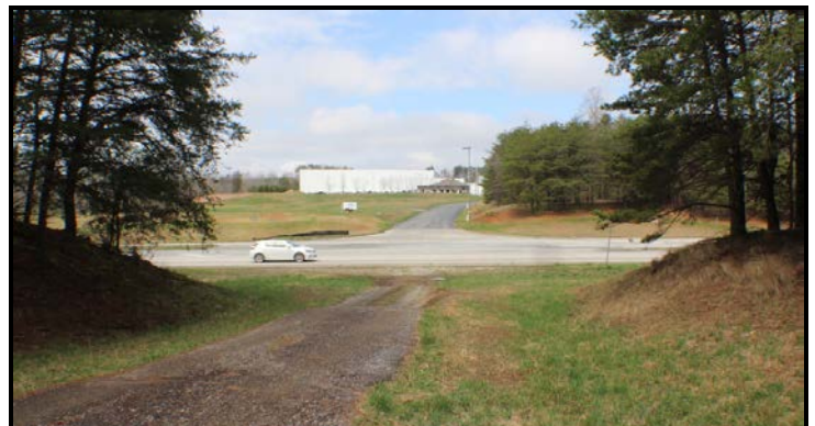
Hwy 365 Entrance with full median break
