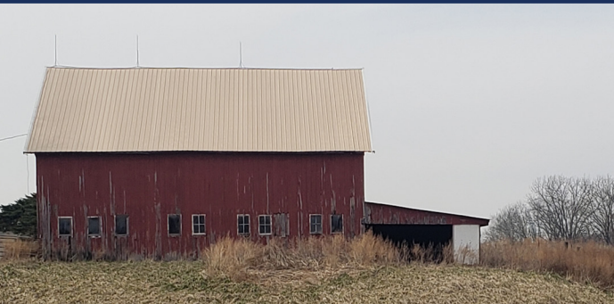
2 Livestock Barns with Concrete Feedlot
