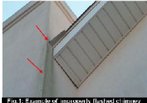
Fig.1: Example of improperly flashed chimney
