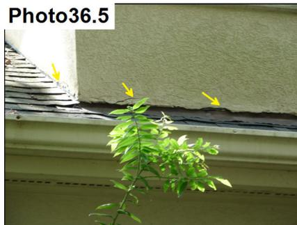
Damaged stucco needs repair.
