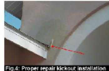
Fig 4: Proper repair kickout installation
