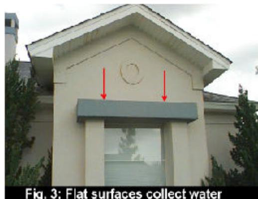
Fig. 3: Flat surfaces collect water
