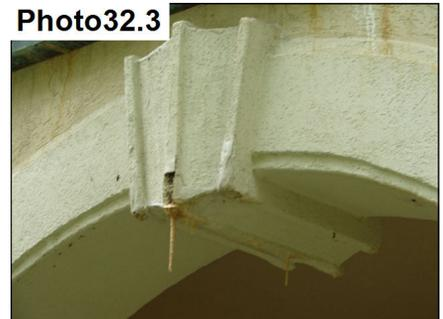
Signs of water entry between the stucco and the concrete construction.
