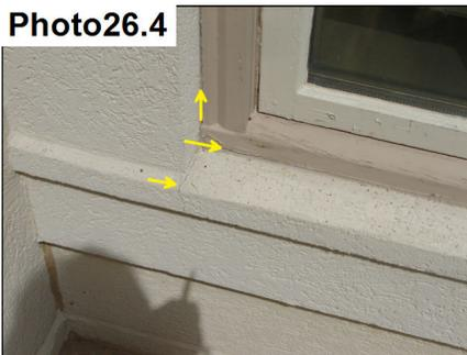
Thin and failing caulk at the window frame, need to re-caulk.
