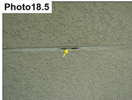
Failed caulked at the joint, need to caulk correctly.
