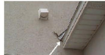
Fig 2: Improper installation (unsealed)
