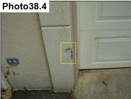
Damaged stucco needs to be repaired.
