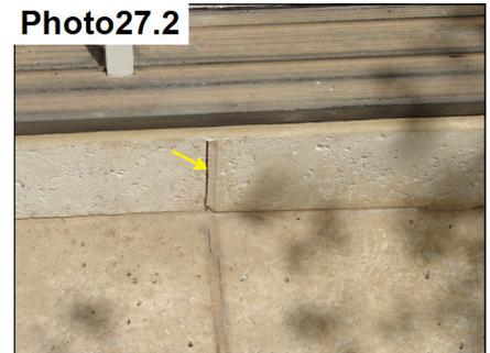
Grout failure, deck area.
