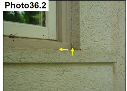
Thin and failing caulk at the window frame, need to re-caulk.
