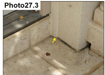
Leak area at deck flowing to lower area.
