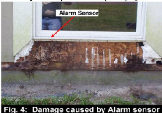
Fig. 4: Damage caused by Alarm sensor
