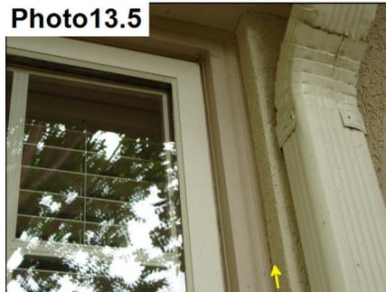
Thin and failing caulk at the window frame, need to re-caulk.
