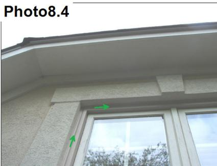
Window caulk at the frame appears to be correct and functioning properly.
