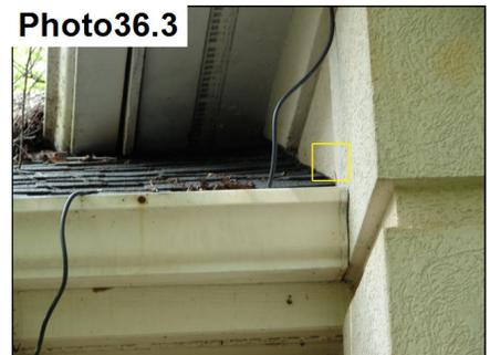
Kickout flashing is missing and needs to be installed.
