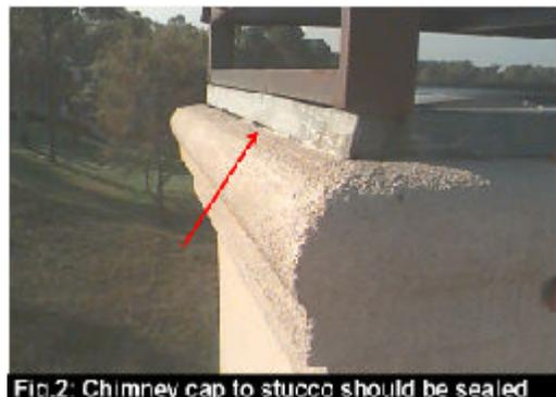
Fig.2: Chimney cap to stucco should be sealed
