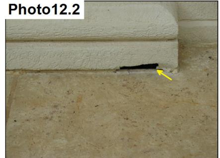
Damaged stucco needs to be repaired/sealed.
