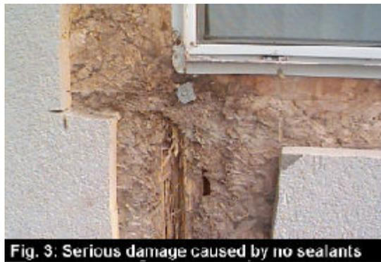
Fig. 3: Serious damage caused by no sealants
