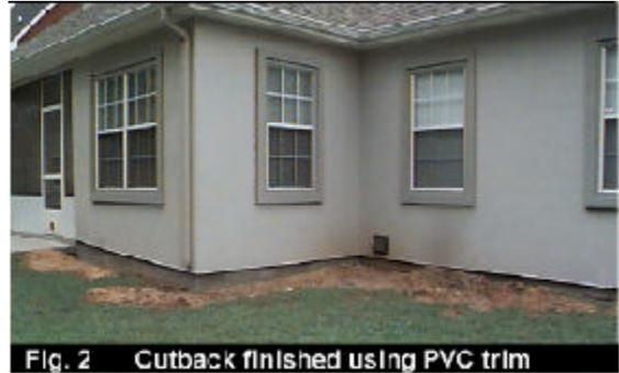
Fig. 2 Cutback finished using PVC trim
