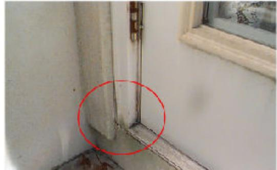
Fig. 1: Damage caused by No sealants
