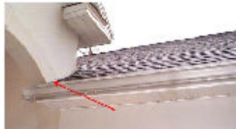
Figure 1: No kickout flashing
