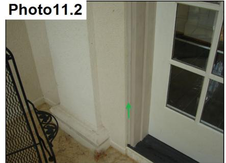
Door frame caulk appears to be correct and functioning properly.
