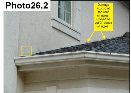
Kickout flashing is missing and needs to be installed.
