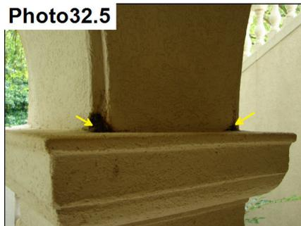
Signs of water entry between the stucco and the concrete construction.
