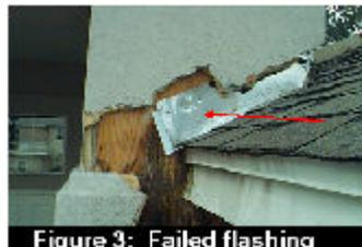
Figure 3: Failed flashing
