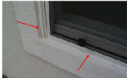
Fig. 2: Example of unsealed window perimeter
