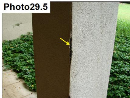
Water entering the stucco between the stucco and concrete.
