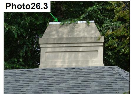
Chimney is capped correctly.
