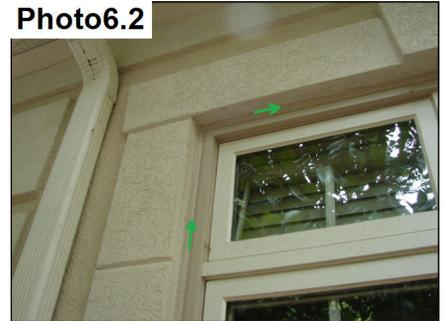
Window caulk at the frame appears to be correct and functioning properly.
