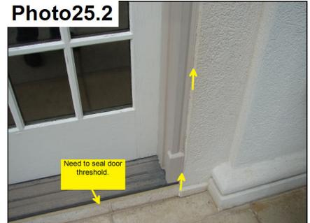
Thin and failing caulk at the door frame, need to re-caulk.
