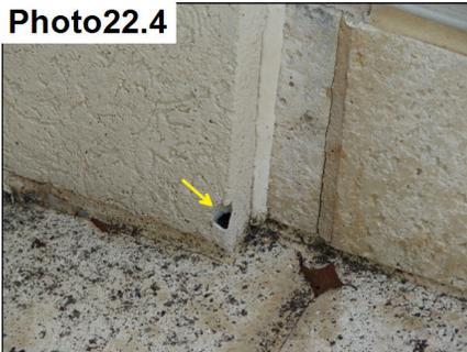
Damaged stucco, need to seal correctly.
