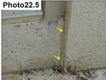
Caulk failure at the accent door threshold area, need to re-caulk.
