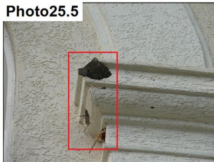
Damaged stucco needs to be repaired.
