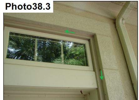
Garage door frame caulk appears to be functioning properly.
