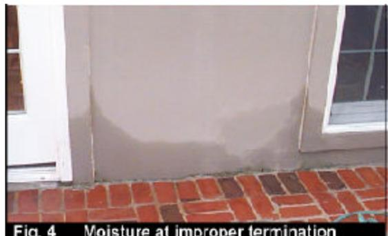
Fig. 4 Moisture at improper termination
