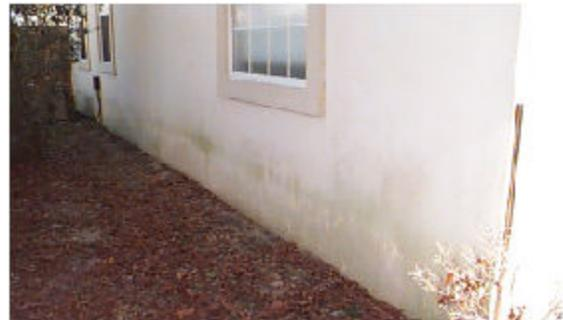
Fig. 1 Moisture caused by the wicking process
