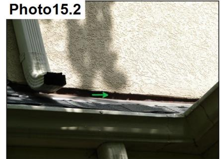
Proper stucco cutback at the roof shingles.
