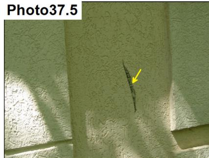
Damaged stucco needs to be sealed.
