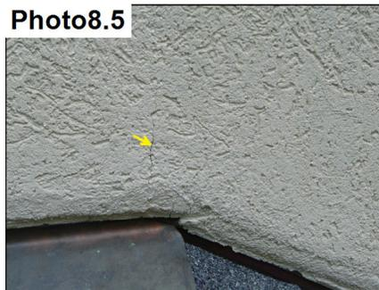
Exposed cracks need to be repaired and or sealed/caulked correctly.
