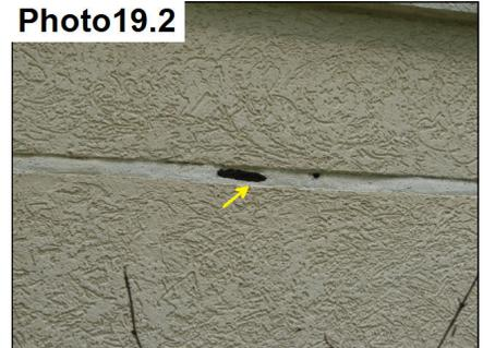
Caulk failure at the joint, need to re-caulk correctly.
