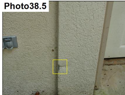
Damaged stucco needs to be repaired.
