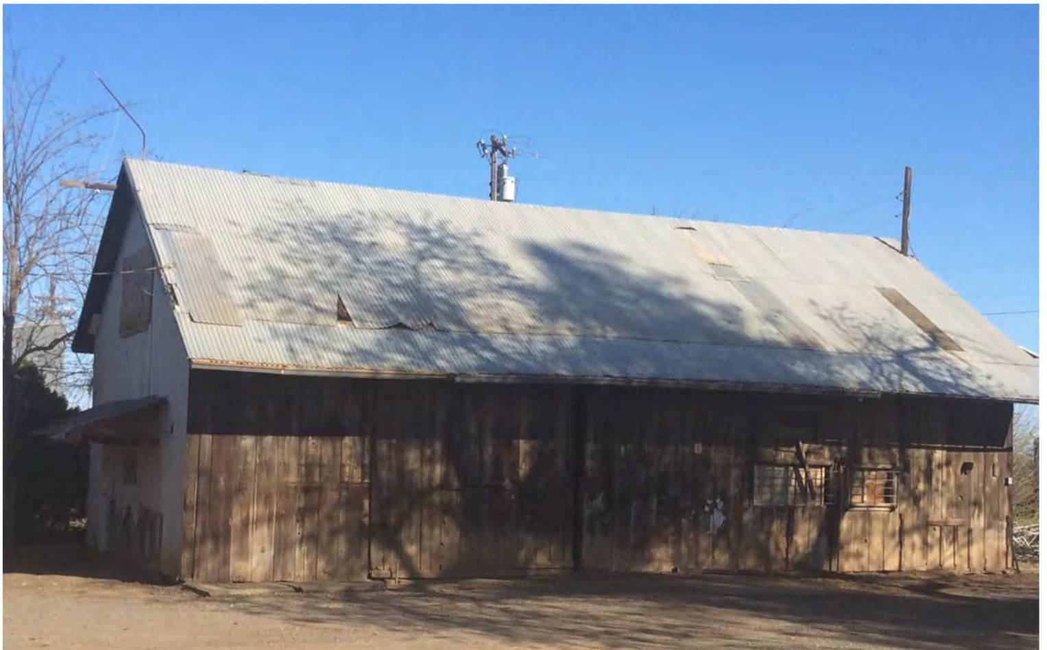
SINGLETON STORAGE BARN #2
