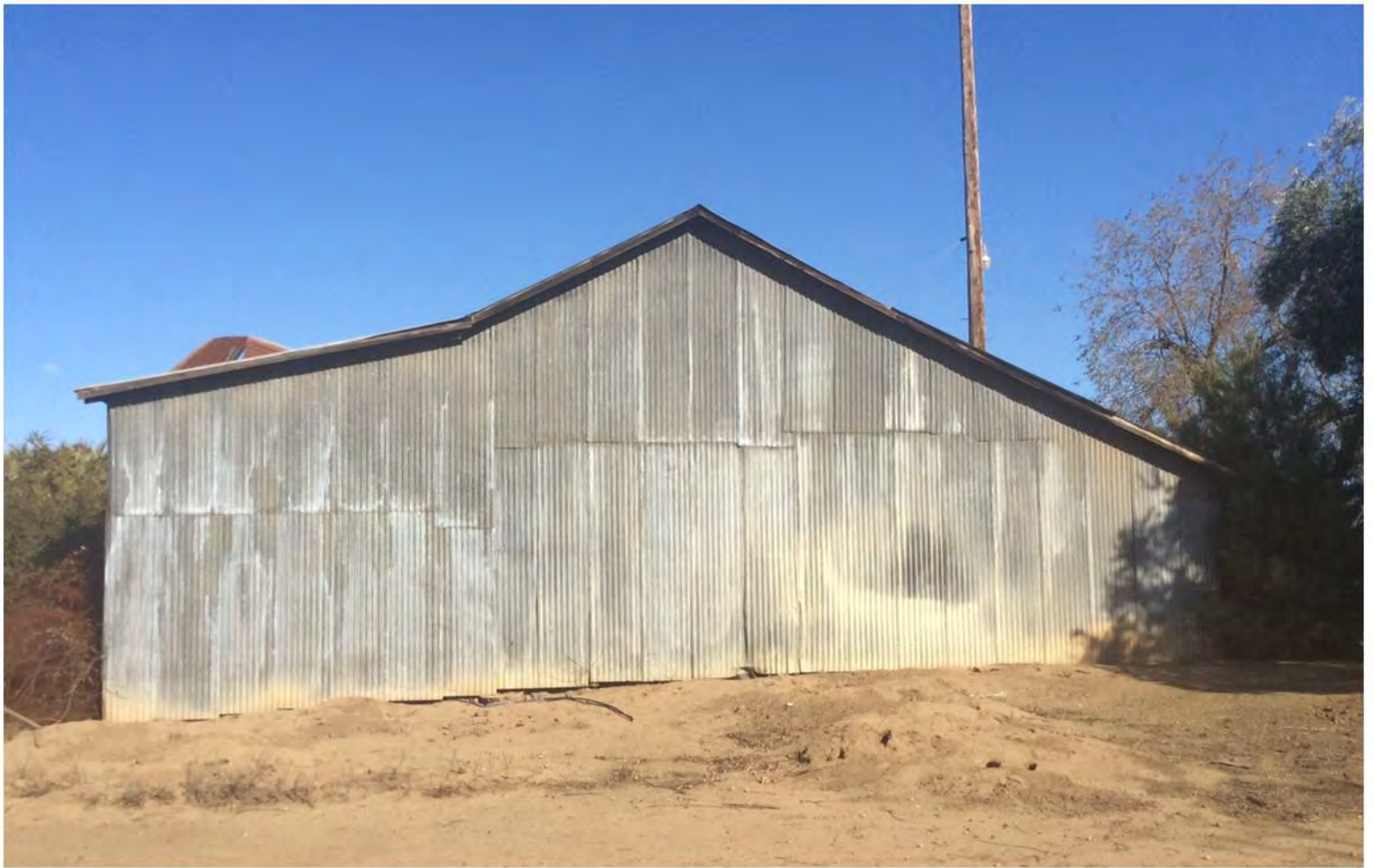
SINGLETON STORAGE BARN #1
