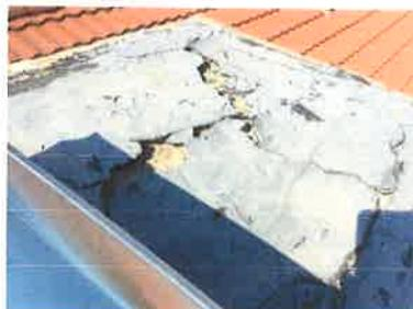
This chimney has the presence of roofing tar, a combustible material, as a sealant. This is dangerous as the temperature around the flue could possibly ignite the tar and start a roof fire. Some of that tar has melted and begun running down the inside of the flue.
