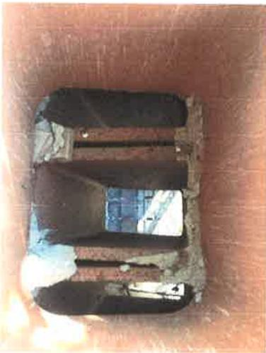
The mortar joints between the flue tiles are no longer intact. These missing or deteriorated mortar joints prevent the flue tiles from properly conveying the byproducts of combustion to the exterior of the home.
