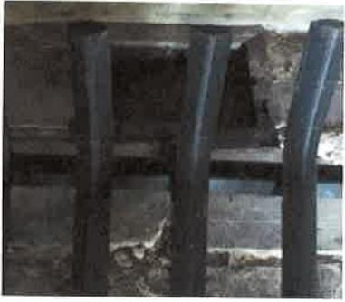
The ash dump door is missing and should be replaced or the ash dump sealed off to prevent hot embers or coals to fall into the ash pit
