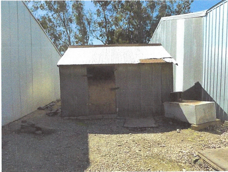
Shed: 16'6" x 12' (198 sq. ft.) shed with concrete slab foundation, wood frame, metal siding and a metal roof.
