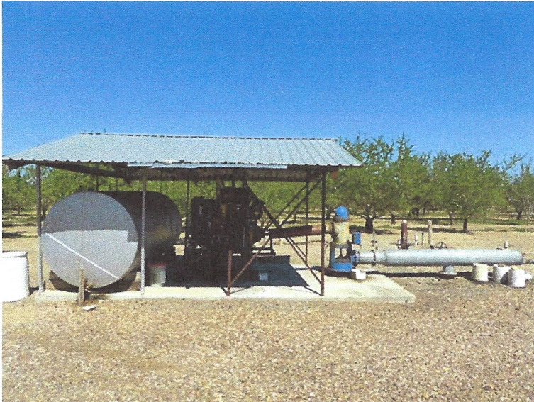
Middle orchard well: CAT Diesel motor Serial No. JKT106904557124 Hours unknown Johnston gear head Serial No. 153253 BJ Turbine Serial No. 816W1586 Morrill Industries sand filter SN 132
