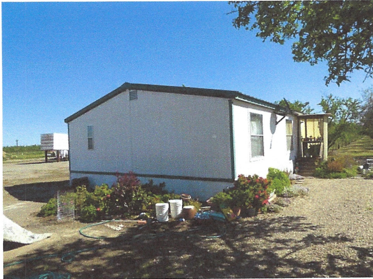
Manufactured home: 27' x 40' (1,080 sq. ft.) home with a perimeter foundation, wood frame, wood siding, and a metal roof.
