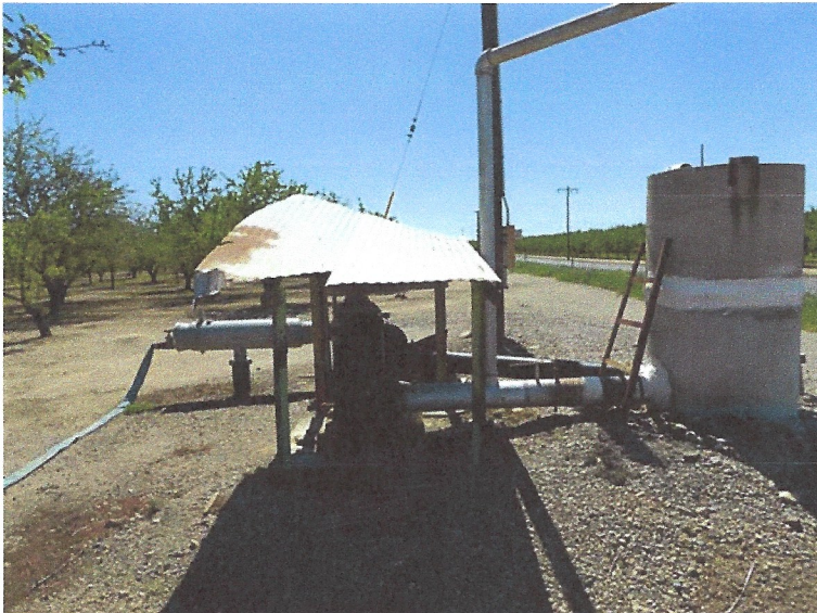
North irrigation well: Pomona Electric motor Serial No. & hp unknown. Morrill Industries sand filter Serial No. 217
