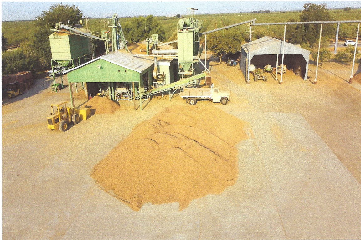
The huller has a Satake Sorter and Forsberg destoner and related huller equipment. The system has approximately 3.33 tons per hour capacity and hulls all the almonds on the property as well as almonds from other growers.
