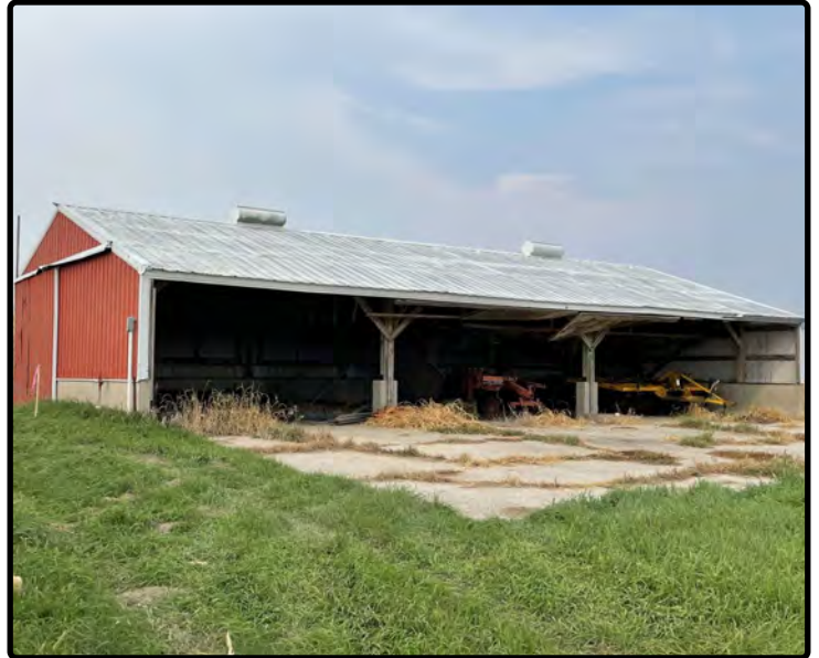
Parcel 4 - Pole Building
