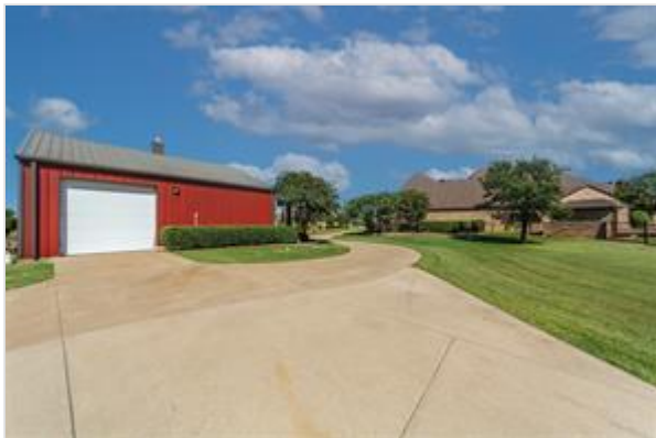
SHOP...Side View Of Building With 10x10 Overhead Door
