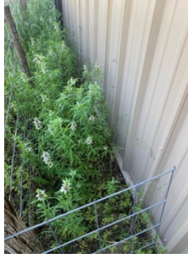
Grading up to the wall on the left side.
