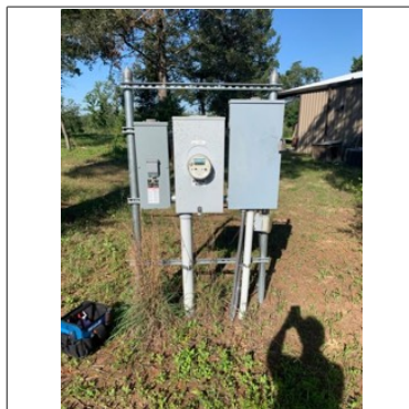
Service entrance is on the right side of building.
