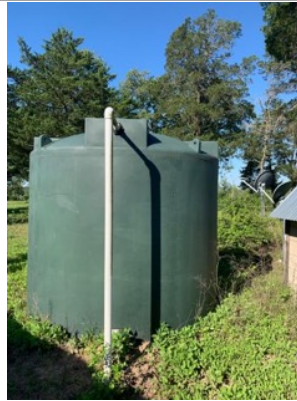
2500 gallon storage tank.
