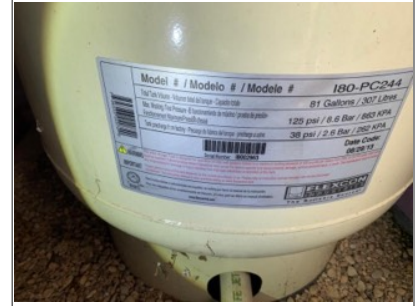
Label on pressurized tank. 81 gallons. Made in 2013.
