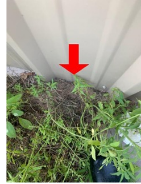
Grading up to wall by left garage door.
