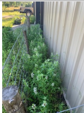
Not all the foundation walls were visible as grading is high.
