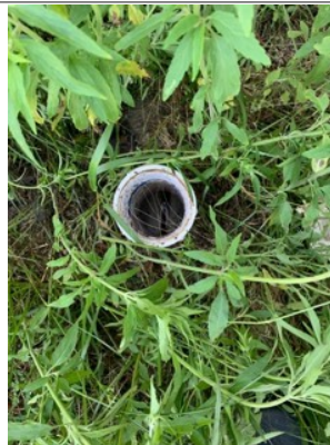
Septic cut-out was clear.
