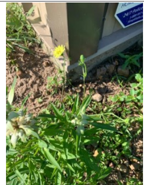
Left rear corner of the foundation.
