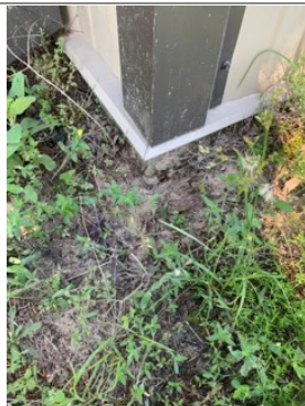
Right rear corner of the foundation.
