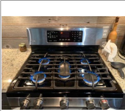
Burners were operational.
