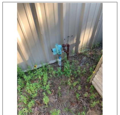
Gas entry is on the right side of the building.
