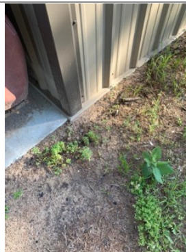
Right front corner of the foundation.
