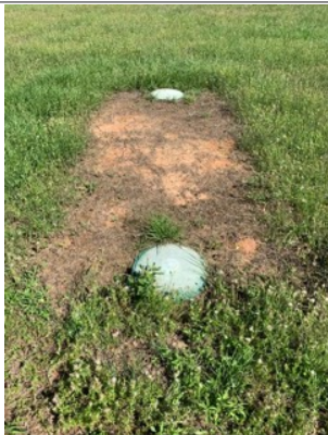
Septic is on the left side of the home. Unable to determine the location of the drain field, or locate any additional equipment to inspect.
