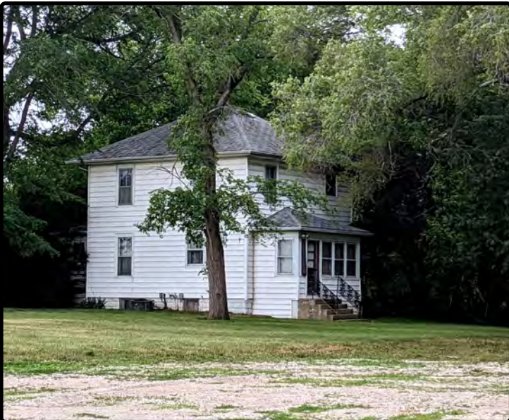
Parcel 9 - Two-Story Farmhouse
