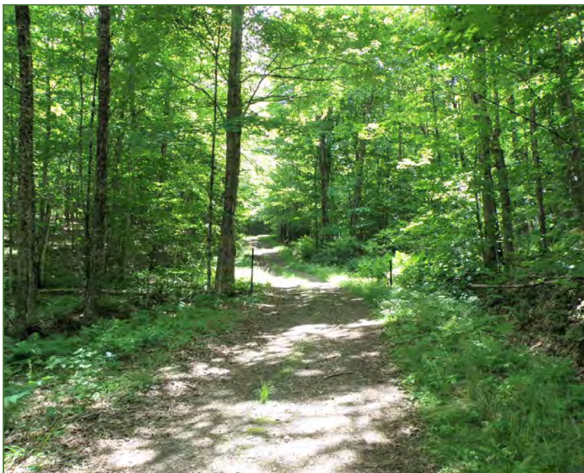
The lower access road as it traverses a maple stand. This gravel road is level with all culverts delineated with iron pipes to facilitate their location and maintenance of cleaning leaf litter from the drainage.
