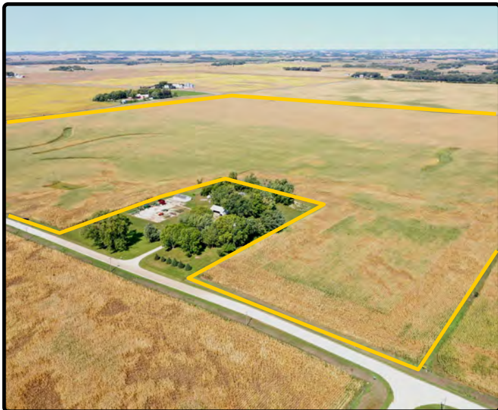
Southeast Looking Northwest
