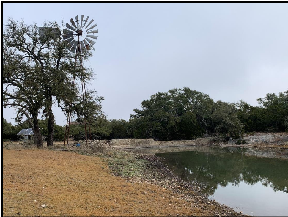
Concrete Dam across Draw Fed by Well with Solar Pump.
