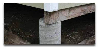
Once piers have cured, forms used for pouring are stripped away. Any nominal space between the top of the pier and the beam is secured with steel shims. Holes are backfilled.
