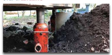
Hydraulic jacks are used to manually level the home under the direction of the Field Superintendent, who monitors the reaction of the structure and interior elevation readings throughout the process.
