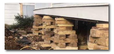
Temporary "shoring" is placed under your home's existing beams. Typically skirting is removed.
