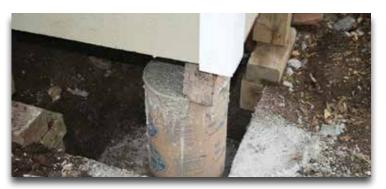
Sonotube forms are cut to span from the top of the previously-poured footing to the new height of the level beam. Concrete is hand-poured into each form.
