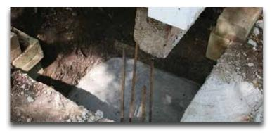
A two-foot by two-foot hole is dug below grade for the footing. Rebar is tied together inside the footing and concrete is poured to a height of 12". Rebar extends up from the center of the pad for pier installation.
