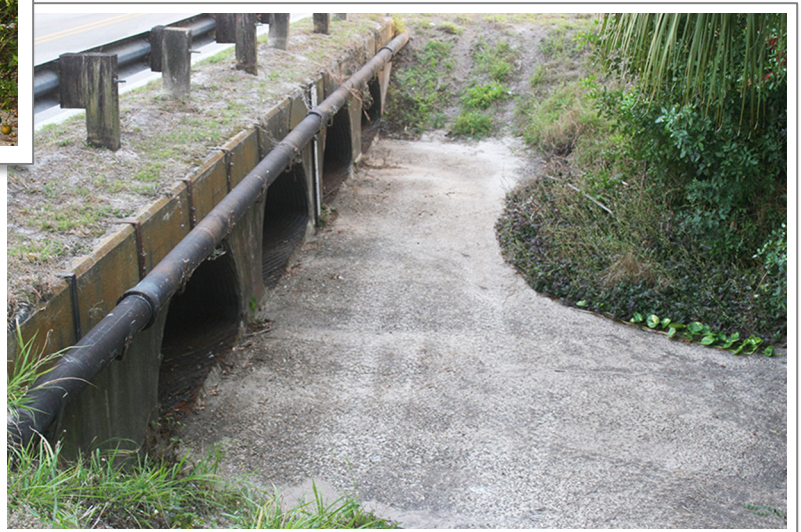
Local Collection Basin and Drainage Culverts
