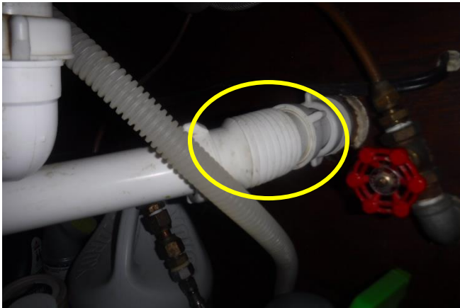
Corrugated drain pipe/Kitchen
