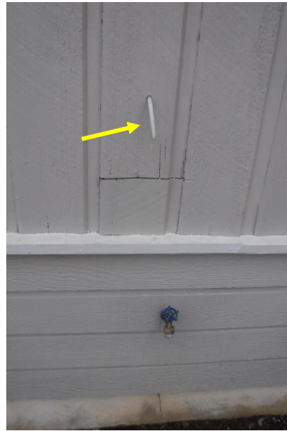
Exterior PRV pipe termination too high
