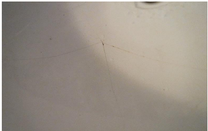
Cracked sink basin/Master bathroom
