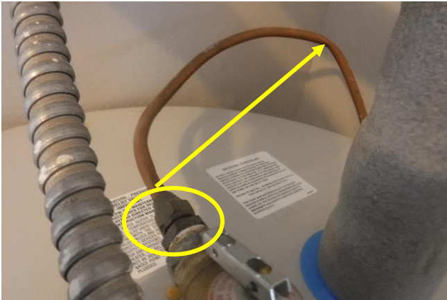
Reduced PRV piping
