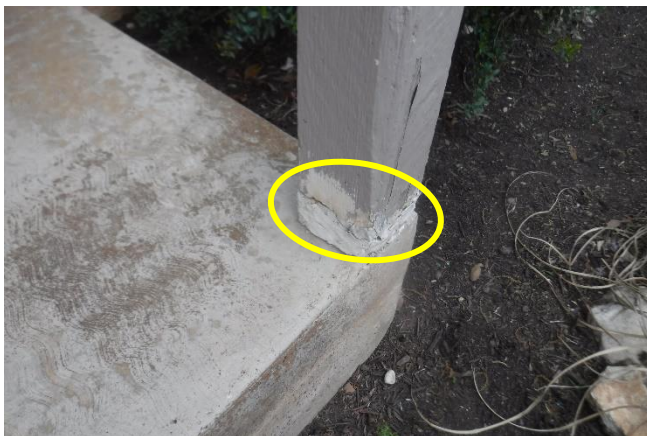
Separated/loose front porch post
