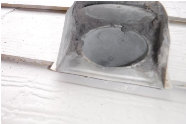
Dryer vent damper
