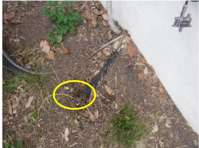
Partially clogged drain pipe
