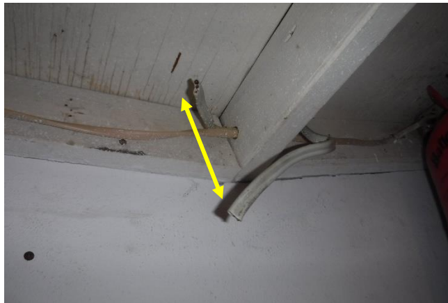
Open wiring/Garage storage area
