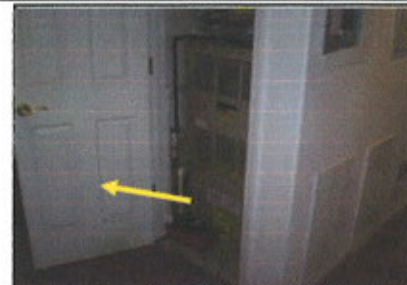
Recommend installation of a louvered door for the furnace closet.
