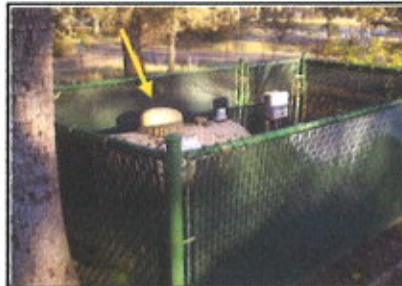
Main gas shut-off is at the tank in the front yard.
