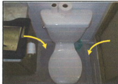
Staining is noted to the floor covering around the toilet & in front of the tub.
