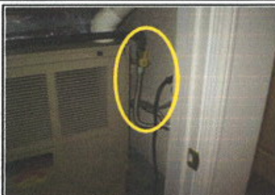
Sediment trap is not installed on the furnace gas supply connector.
