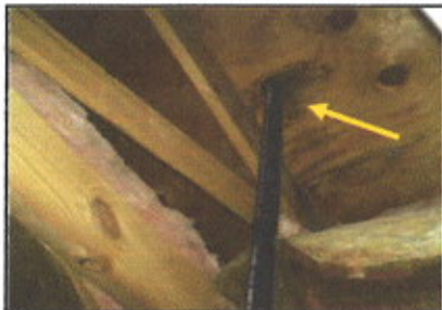
Staining is noted at the upper plumbing vent pipe entry through the roofing.
