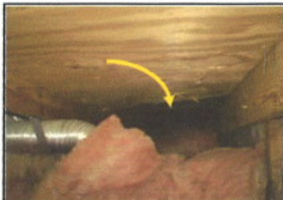
Moisture buildup & black staining is noted at the master bathroom exhaust discharge.
