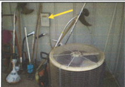
AC condenser &amp; in-sight disconnect.
