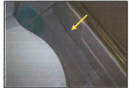
Lifting is noted to the floor covering along the front of the tub.
