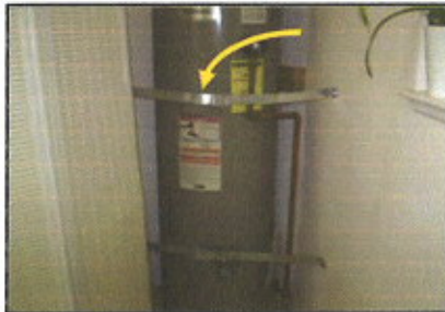
EQ strapping is loose, not securing the water heater from movement.
