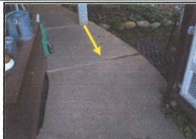
Uplifted edges are noted in the side walkway.
