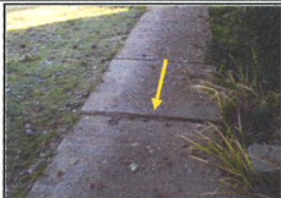
Uplifted edges are noted in the front walkway.
