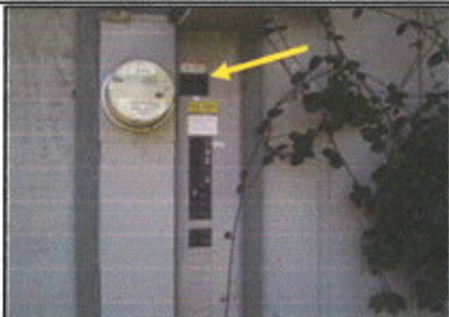
House main electrical service entrance & disconnect breaker.
