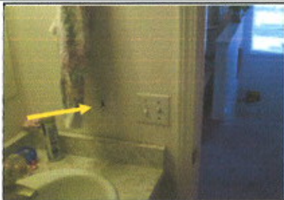
GFCI reset for the exterior & bathrooms outlets in in the upper half bathroom.
