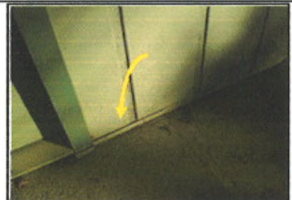
Unsealed pan flashing will allow water to trap behind the flashing.
