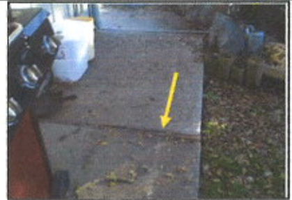
Uplifted edges are noted in the rear walkway.
