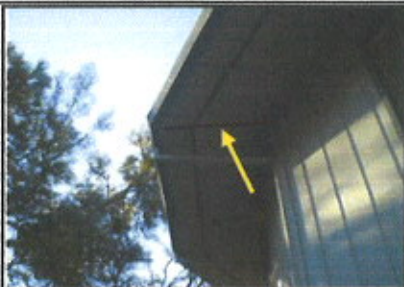
Loose trim material is noted under the eave soffits around the house.
