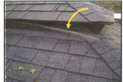
Loose vent screen at the roof cupola over the garage may allow animal entry into the garage attic.
