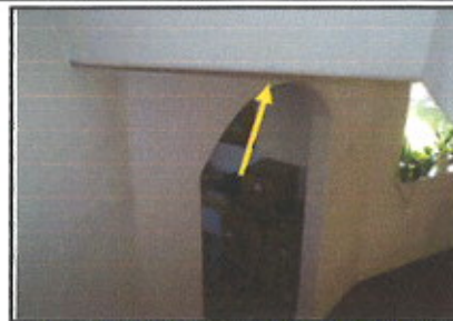
Low head clearance is noted at the bottom of the stairs.
