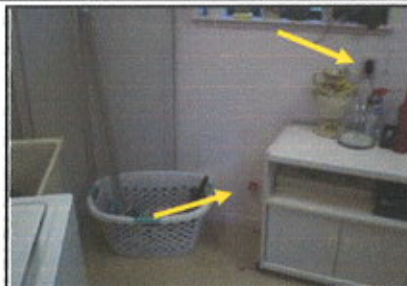
Wall outlets located within 6 ft of the laundry sink are not GFCI protected.
