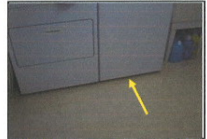
Drain/ catch pan is recommended under interior installed washers.
