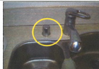
Water noted discharging out of the air gap device indicates debris in the dishwasher drain line hose.
