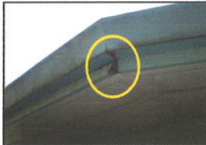
Rusting/leaking is noted at multiple gutter joints.
