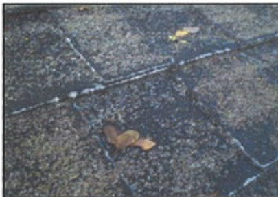
Roofing shingles are reaching their expected life.
