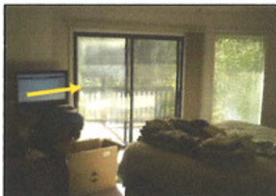
Master bedroom - failed thermo seal/fogging is noted in the slider door.
