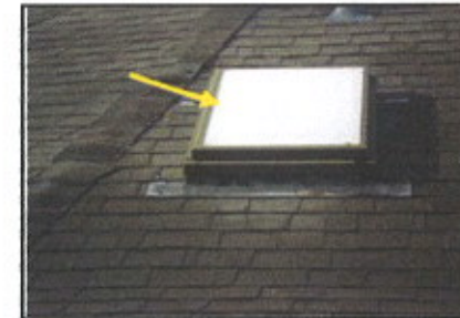
Master bedroom skylight cover is cracked.
