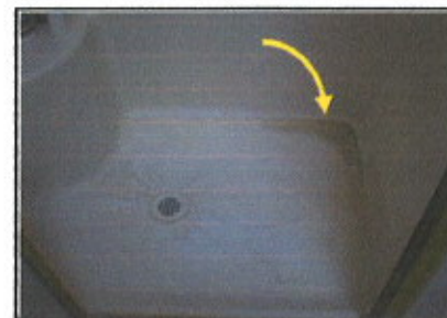
Water ponds in the right rear corner of the shower pan.
