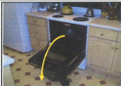
Anti-tip bracket is not installed for the oven/ stove.
