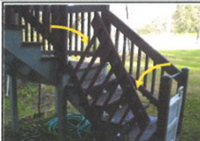
Bottom steps railing is detached from the post.
