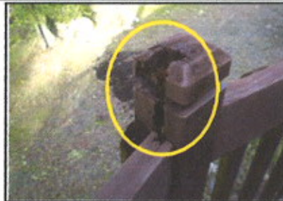
Deterioration is noted to the deck & deck steps railings & posts material.
