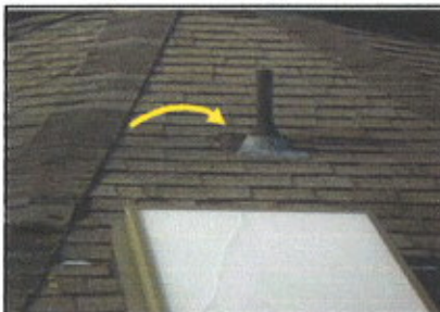
Staining/water entry is noted at the upper plumbing vent pipe roof penetration.
