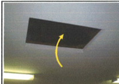
Attic access opening in the garage ceiling reduces the garage to house fire protection.
