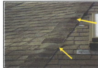
Loose & missing shingles are noted.
