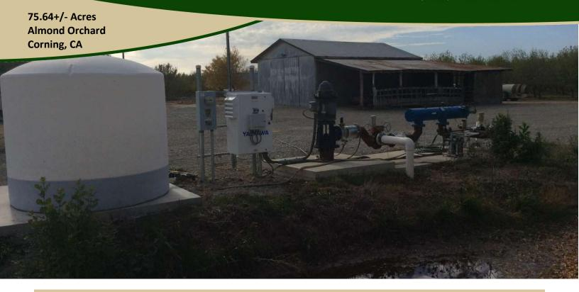
Well, Filter, Fertilizer Injection System, and Wiseconn Remote Technology
