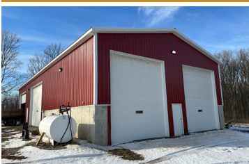
40' x 80' Machinery Shed with (4) overhead doors, concrete floor, 4' concrete side walls.
