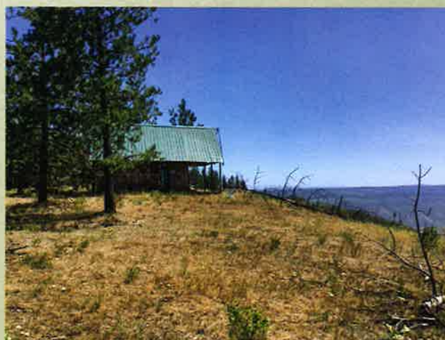
Second cabin requires some repair
