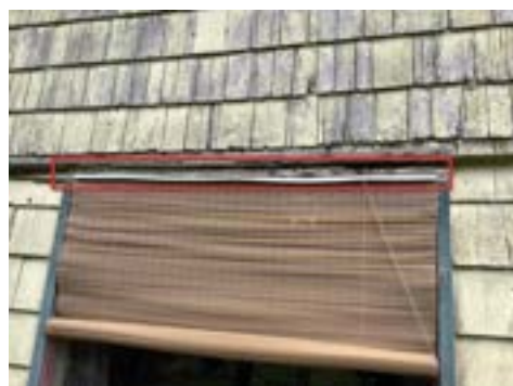
Siding/Trim Wood Rot (Representative Picture)
