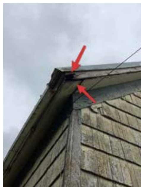
Fascia/Eave Wood Rot (Representative Picture)
