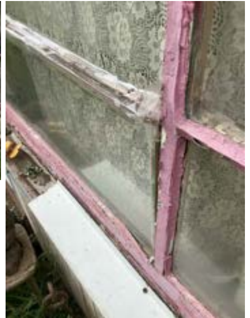
Window Trim/Frame Wood Rot (Representative Picture)
