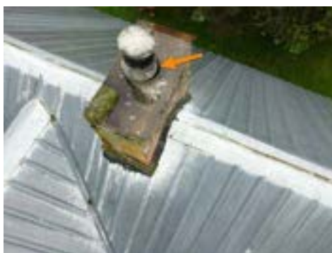
Gap Around Vent Stack - Center Ridgeline
