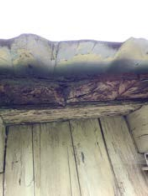
Roof Decking Wood Rot (Representative Picture)
