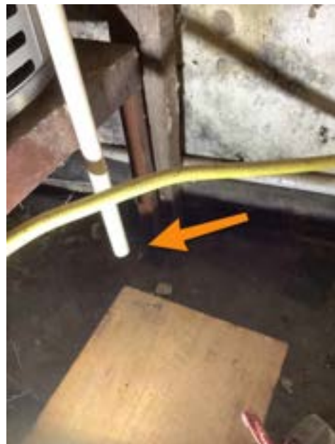
TPR Valve Discharges Onto Floor - Utility Room (First Floor)
