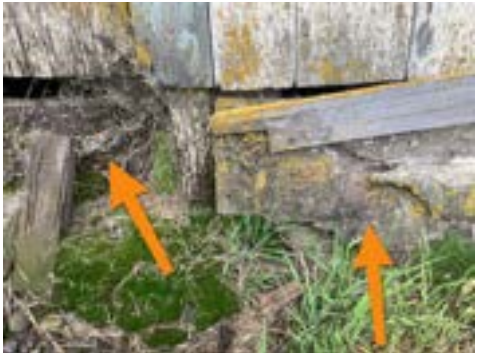
Skirting Wood Rot (Representative Picture)
