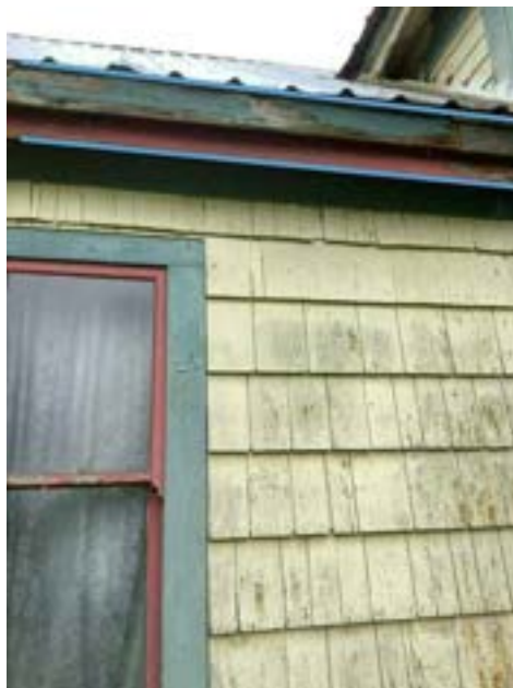
Fascia/Eave Paint Deteriorating (Representative Picture)
