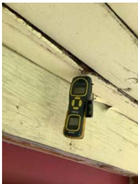
Fascia/Eave Wood Rot (Representative Picture)
