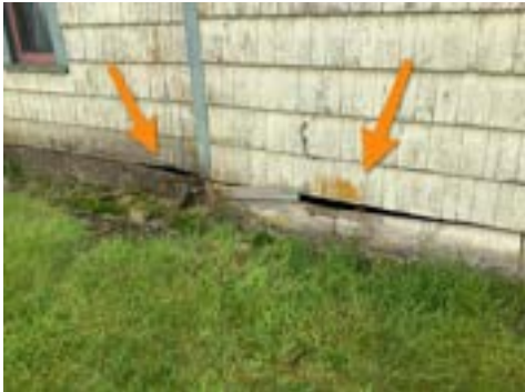
Skirting Wood Rot (Representative Picture)
