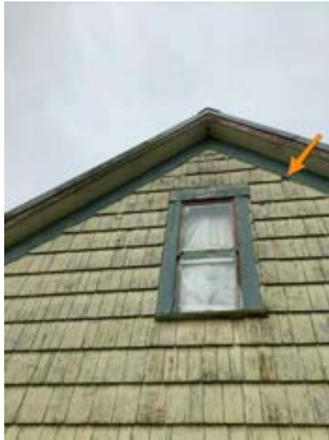
Section(s) of Missing Siding (Representative Picture)
