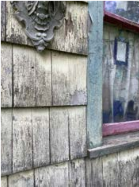
Siding/Trim Paint Deteriorating (Representative Picture)
