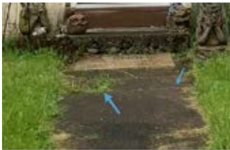
Walkway Crack(s) - Side A (Representative Picture)
