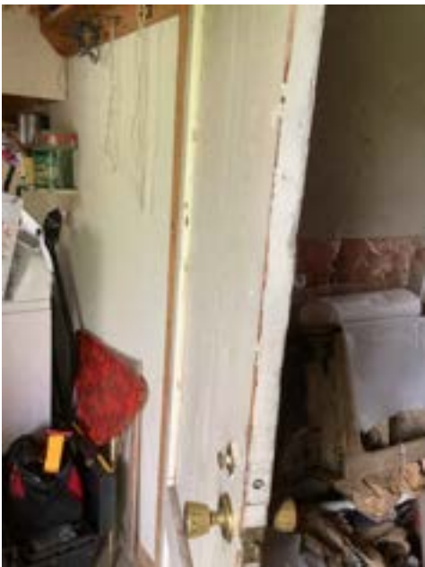
Door Does Not Meet Separation Requirements - Garage
