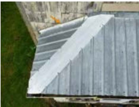
Siding in Contact With Roof (Representative Picture)
