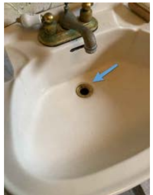
Drain Stop Missing - Full Bathroom (First Floor)
