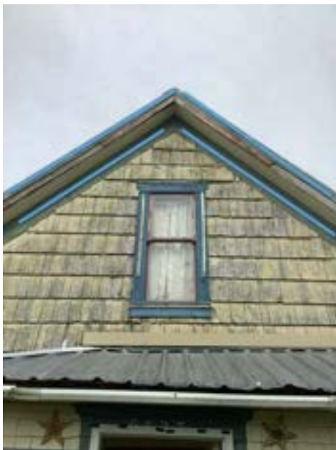
Fascia/Eave Paint Deteriorating (Representative Picture)
