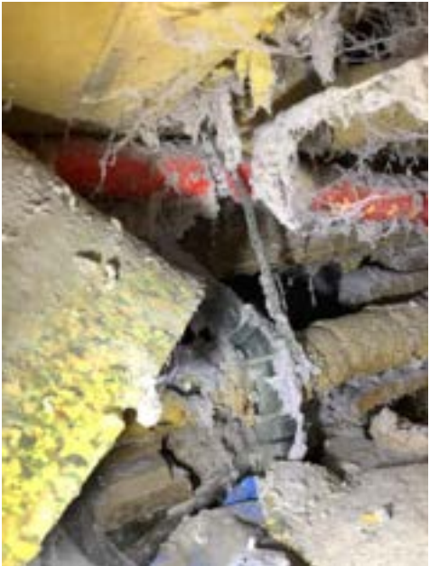
Dryer Exhaust Improperly Venting - Crawl Space
