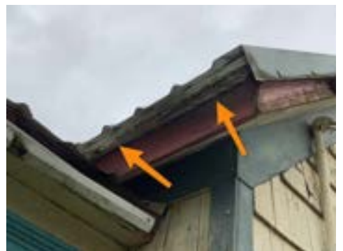
Multiple Roofing Layers (Representative Picture)
