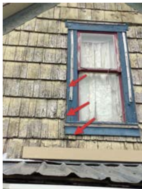
Siding/Trim Wood Rot (Representative Picture)
