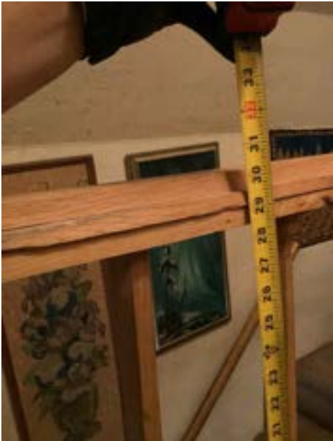
Insufficient Height of Guardrail - Hallway (Second Floor)
