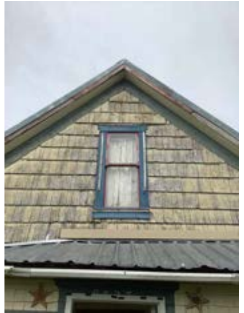
Siding/Trim Paint Deteriorating (Representative Picture)
