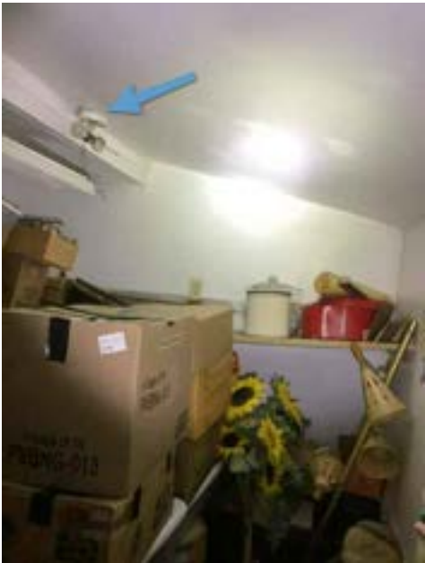
Light Fixture Cover Missing - Garage
