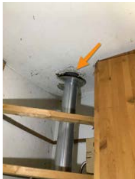
Ceiling Damaged - Utility Room (First Floor)
