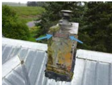
Chimney Mortar Deteriorating - Center Ridgeline
