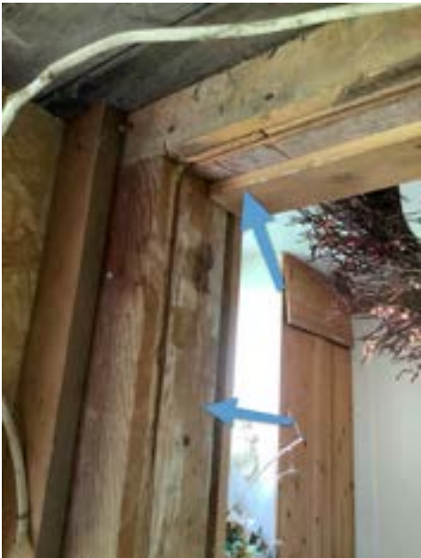
Weather-Stripping Not Present - Garage
