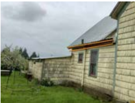
Gutter System Damaged/Not Present (Representative Picture)
