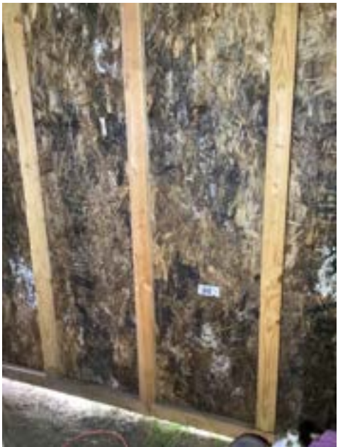
Garage Door Wood Rot - Side B (Representative Picture)
