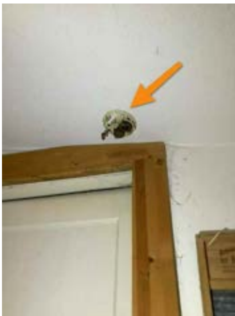
Smoke Detector(s) Damaged (Representative Picture)
