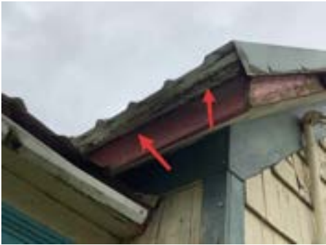
Roof Decking Wood Rot (Representative Picture)
