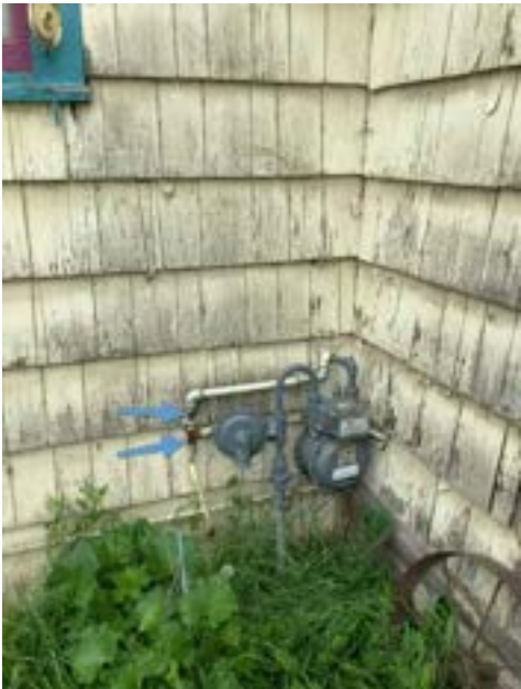
Corroded Gas Supply Line - Side B
