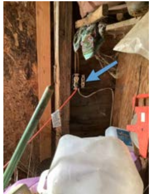
Outlet Cover Plate Missing - Garage
