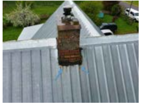
Corroded Roof Covering (Representative Picture)
