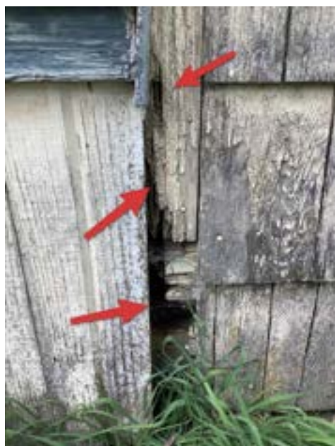
Siding/Trim Wood Rot (Representative Picture)
