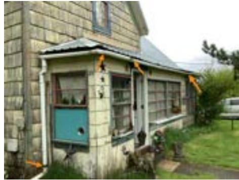
Gutter System Damaged/Not Present (Representative Picture)
