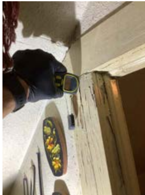
Signs of Moisture Damage - Bedroom (Second Floor)
