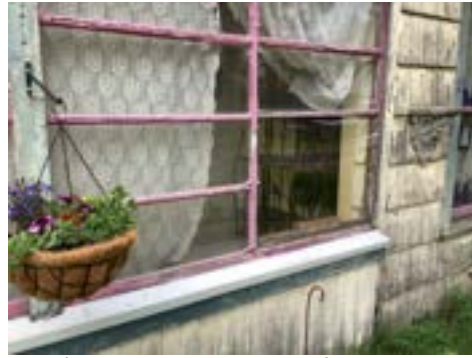
Window Trim/Frame Wood Rot (Representative Picture)
