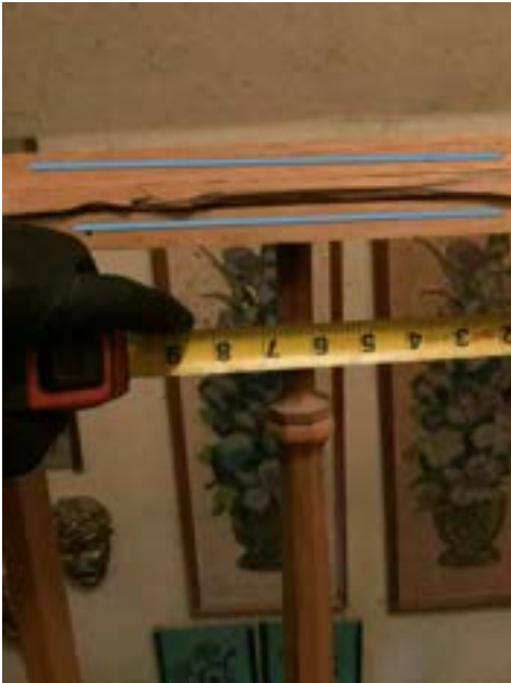
Guardrail Damaged - Hallway (Second Floor)
