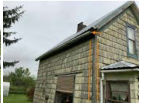
Gutter System Damaged/Not Present (Representative Picture)
