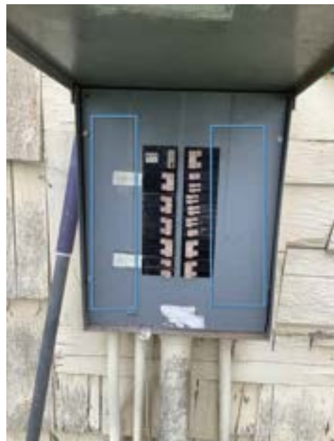
Insufficient Labeling of Electrical Panel - Side B
