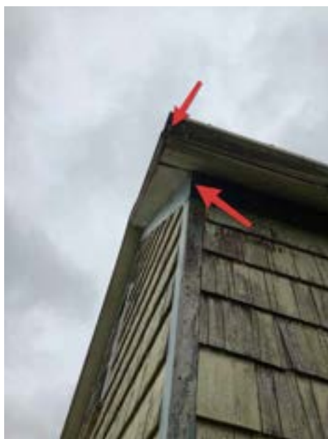
Fascia/Eave Wood Rot (Representative Picture)
