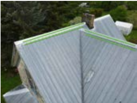
Ridge Vent(s) (Representative Picture)
