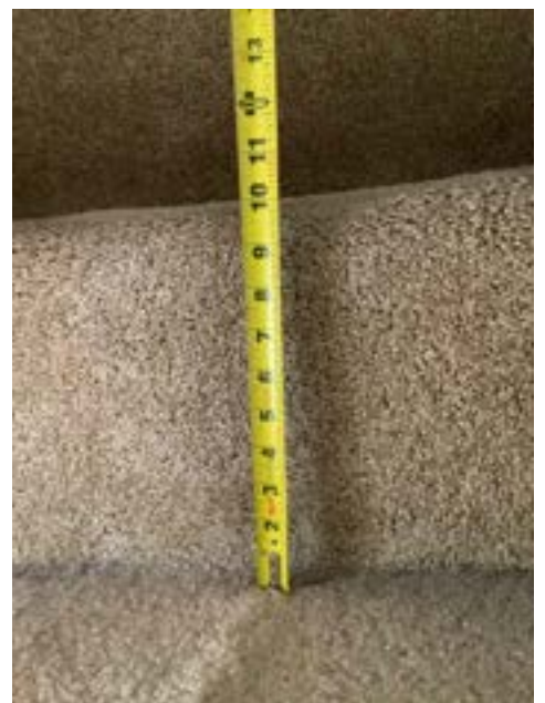
Step Riser(s) Exceed Recommended Height - Stairway (First Floor to Second Floor) (Representative Picture)
