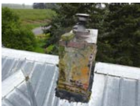
Moss Growth on Chimney Structure - Center Ridgeline (Representative Picture)
