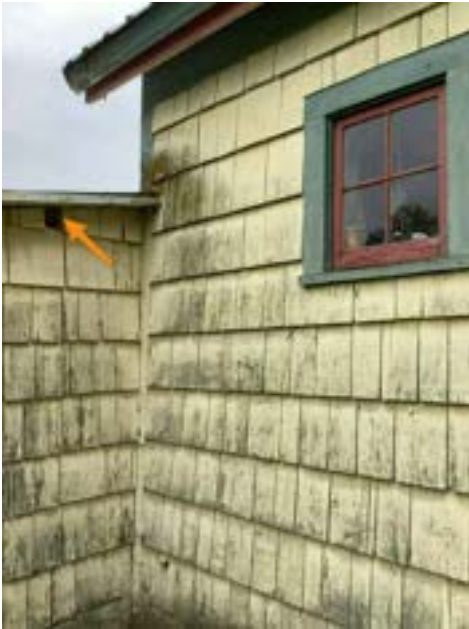
Section(s) of Missing Siding (Representative Picture)
