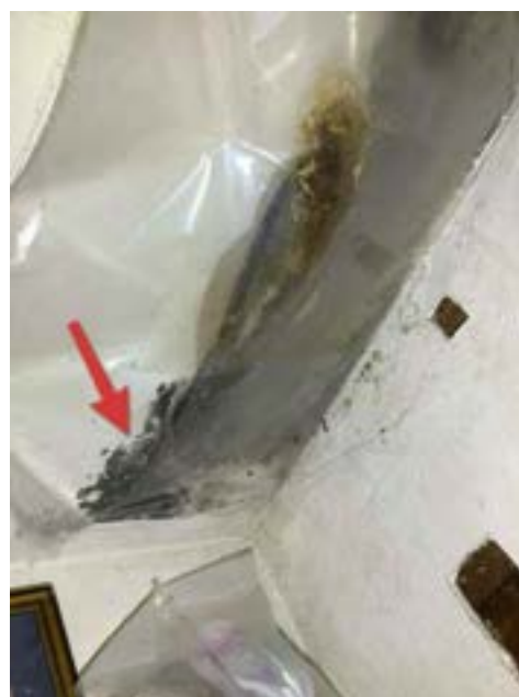
Signs of Possible Microbial Growth - Bedroom (First Floor - On Right)
