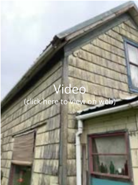
Gutter System Damaged/Not Present (Representative Picture)
