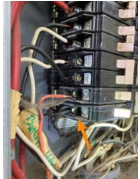
Breaker #23 Incorrectly Wired - Side B
