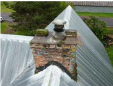
Chimney Mortar Deteriorating - Center Ridgeline
