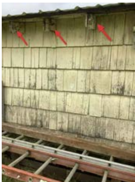
Rafter Wood Rot (Representative Picture)
