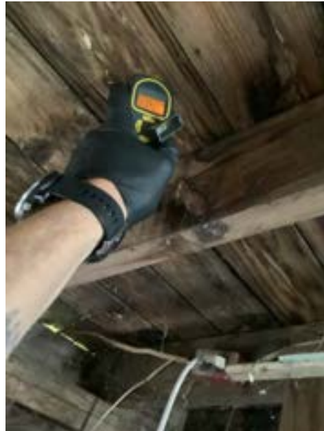
Ceiling Structure Wood Rot - Garage (Representative Picture)
