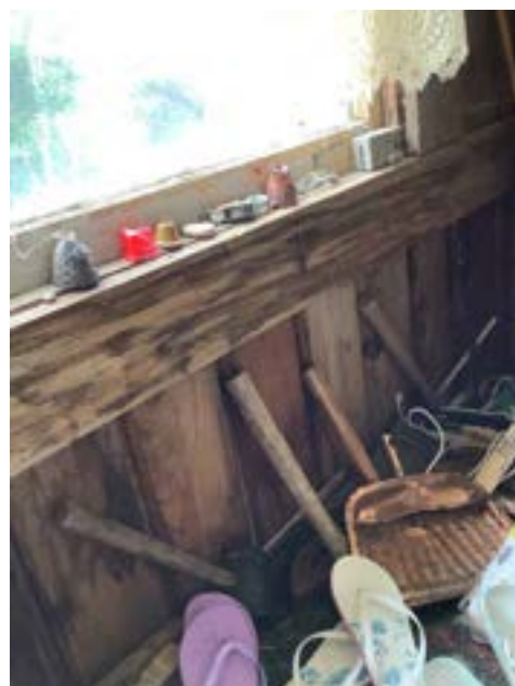
Siding/Trim Wood Rot (Representative Picture)
