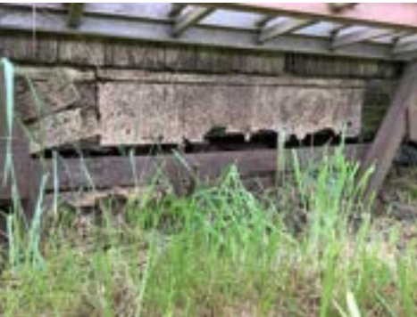
Skirting Wood Rot (Representative Picture)
