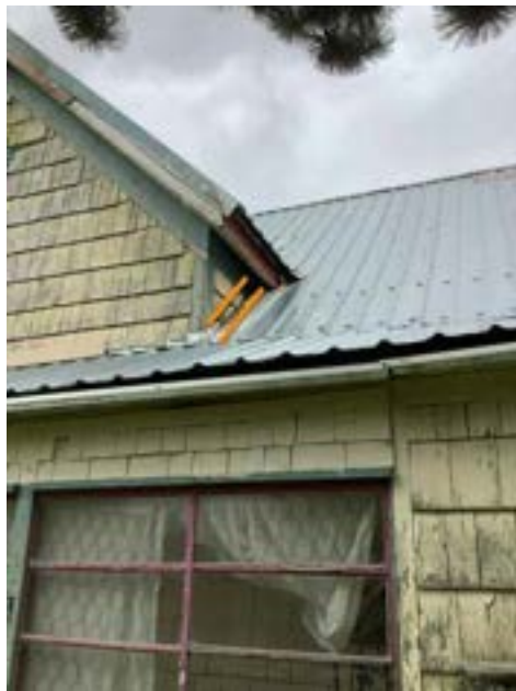
Siding in Contact With Roof (Representative Picture)
