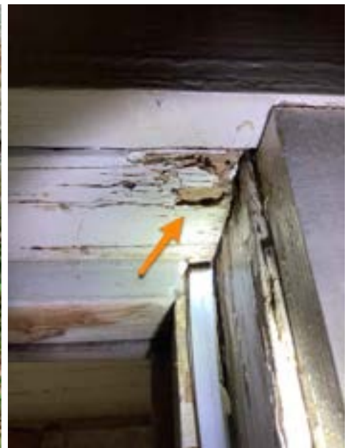
Signs of Wood Destroying Insects (Representative Picture)
