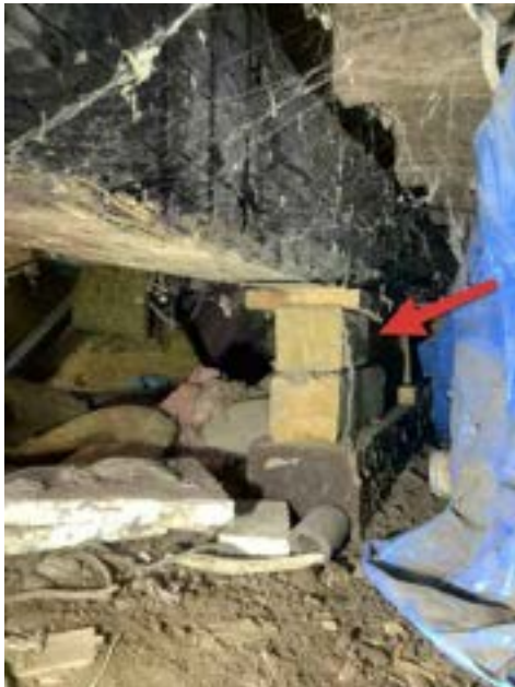
Floor Structure Improperly Braced - Crawl Space (Representative Picture)
