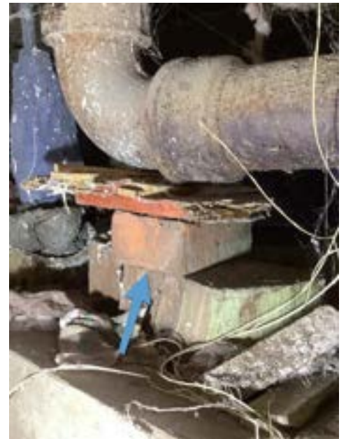
Improperly Supported Drain/Waste Piping - Crawl Space
