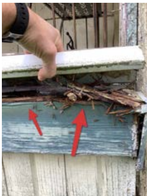
Siding/Trim Wood Rot (Representative Picture)
