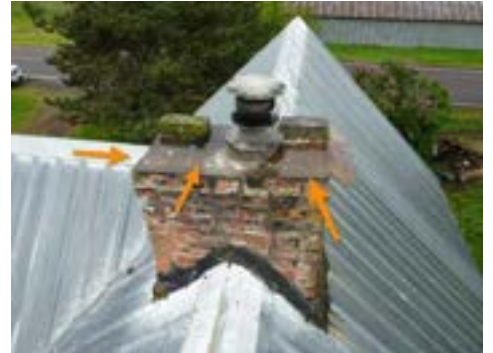
Corroded Chimney Crown - Center Ridgeline
