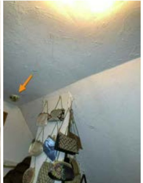
Smoke Detector(s) Damaged (Representative Picture)
