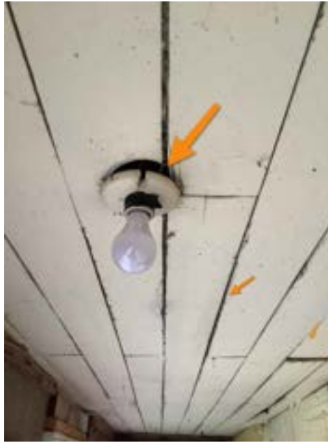
Picture 1b - Eave Panel Gaps (Representative Picture)
