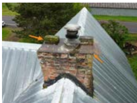
Chimney Crown Not Properly Installed - Center Ridgeline
