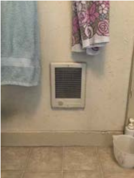
Electric Wall Heater(s) (Representative Picture)
