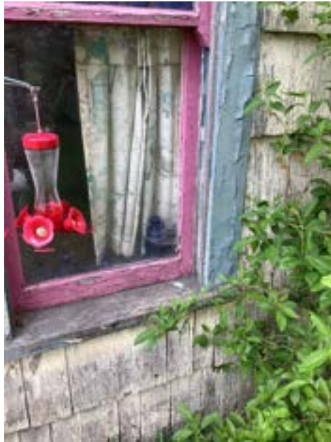
Siding/Trim Paint Deteriorating (Representative Picture)
