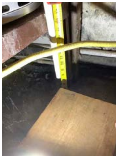
Incorrect Length of TPR Valve Piping - Utility Room (First Floor)
