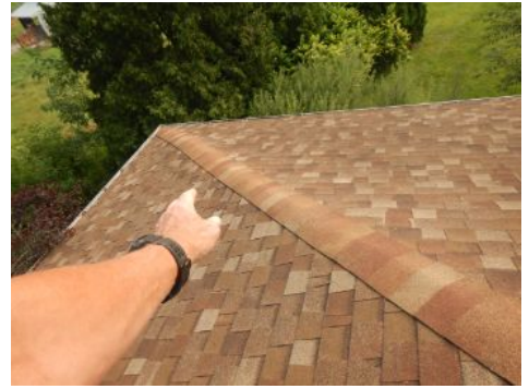
somewhat wavy (likely built this way as no signs of any structural failures)
