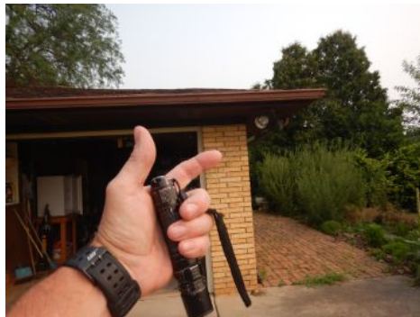
Light did not function at time of inspection
