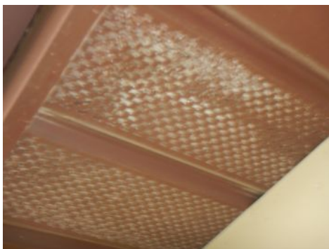
soffit stains/ oxidation above bump out
