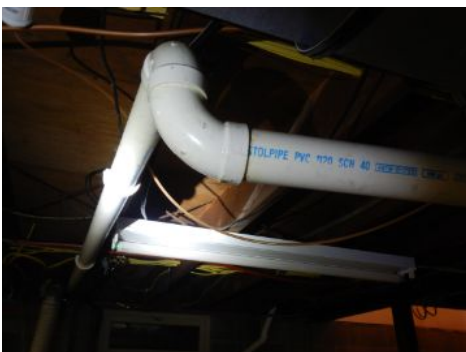
some drains leave basement at floor. some leave elevated
