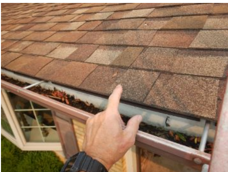
One visible layer of asphalt shingles
