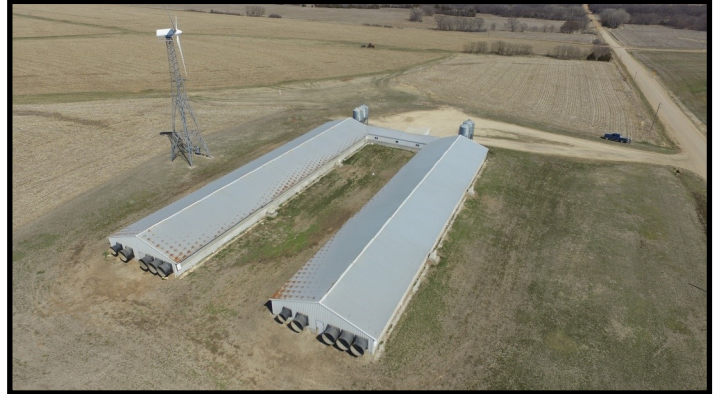
View of Site from the Southwest
