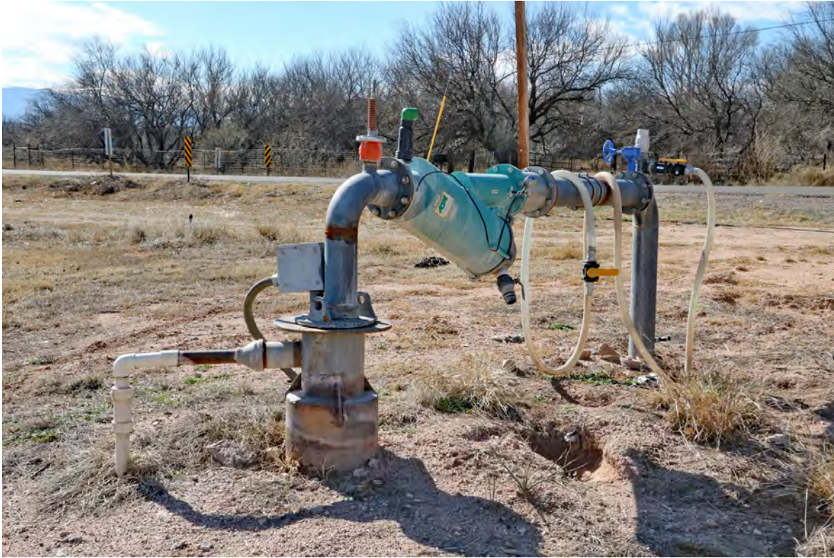
Primary well; 1,286 foot depth, 12 inch casing with 75 hp electric submersible pump.
