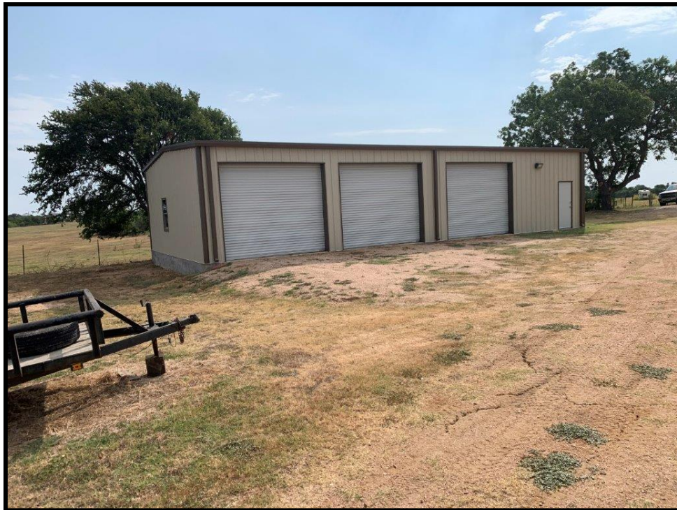
Recent Constructed 1,800 SF Metal Building.
