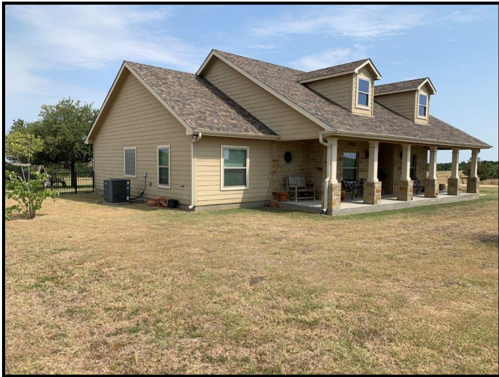
Front View Of Residence.
