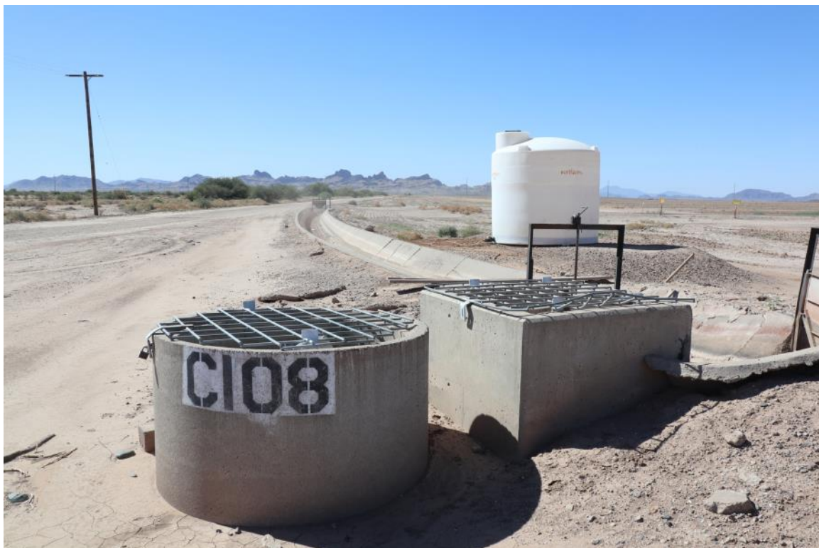
Irrigation district turn-out, CAIDD C108
